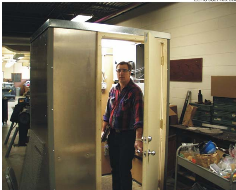
Figure 5. Exterior control room with interior visible through doorway.
