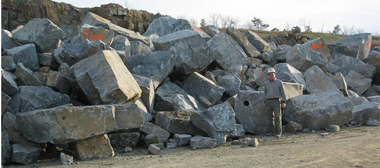
Figure 27. Oversize rocks from the MTM blast that have been set aside.
