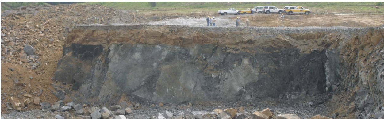
Figure 4. Easterly view of Blast 2904 with blasted muck pile to the left.
