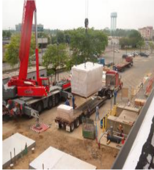
Rigging fuel cells onto concrete pads
