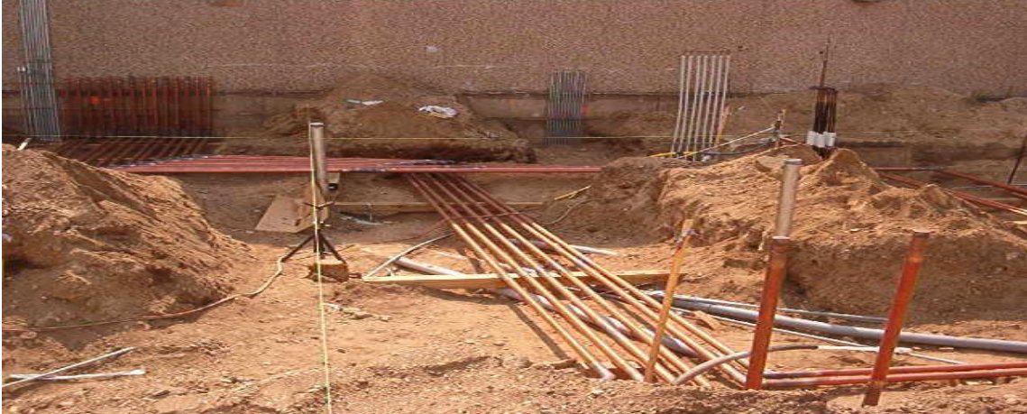
subterranean piping installation
