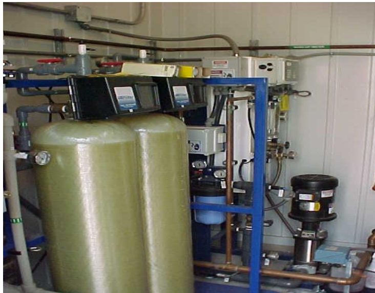
Reverse Osmosis system to fuel cells
