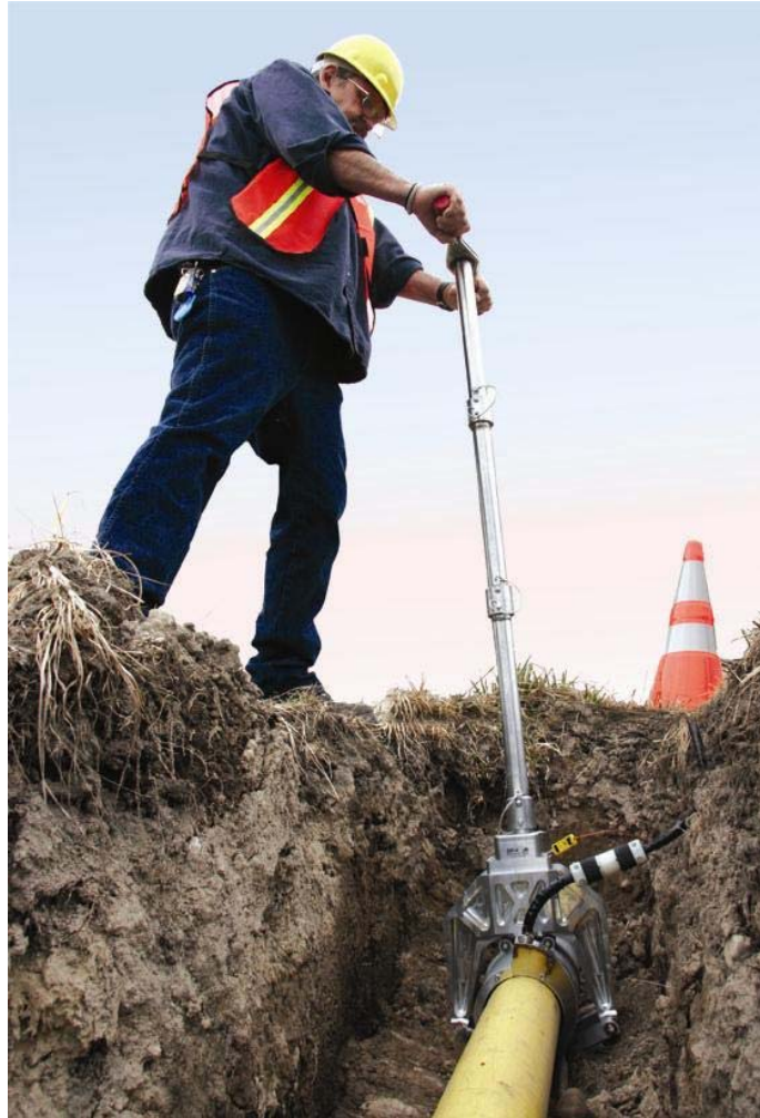
Figure 52: Final engineered prototype applying a PE gel film patch on 4-inch MDPE pipe
