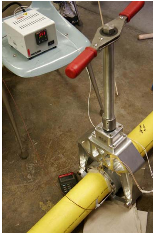
Figure 14: Test tool successful in bonding the repair patch to 4-inch PE pipe
