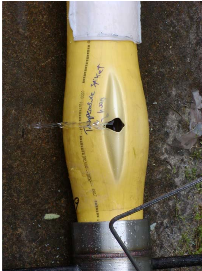
Figure 26: Quick burst test shows pipe failure below PE gel film patch – Indicative of successful bonding
