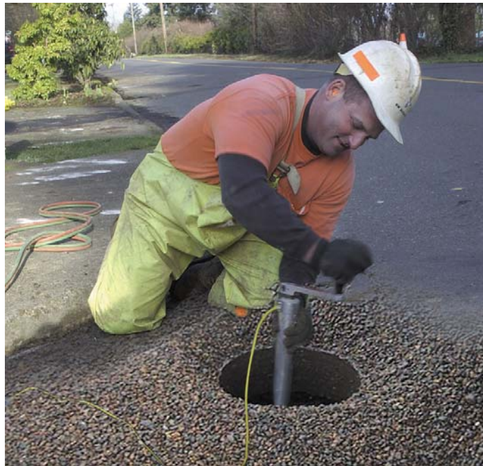
Figure 1: Keyhole Excavation
