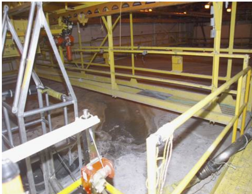
Figure 5. Grouted South Basin.
