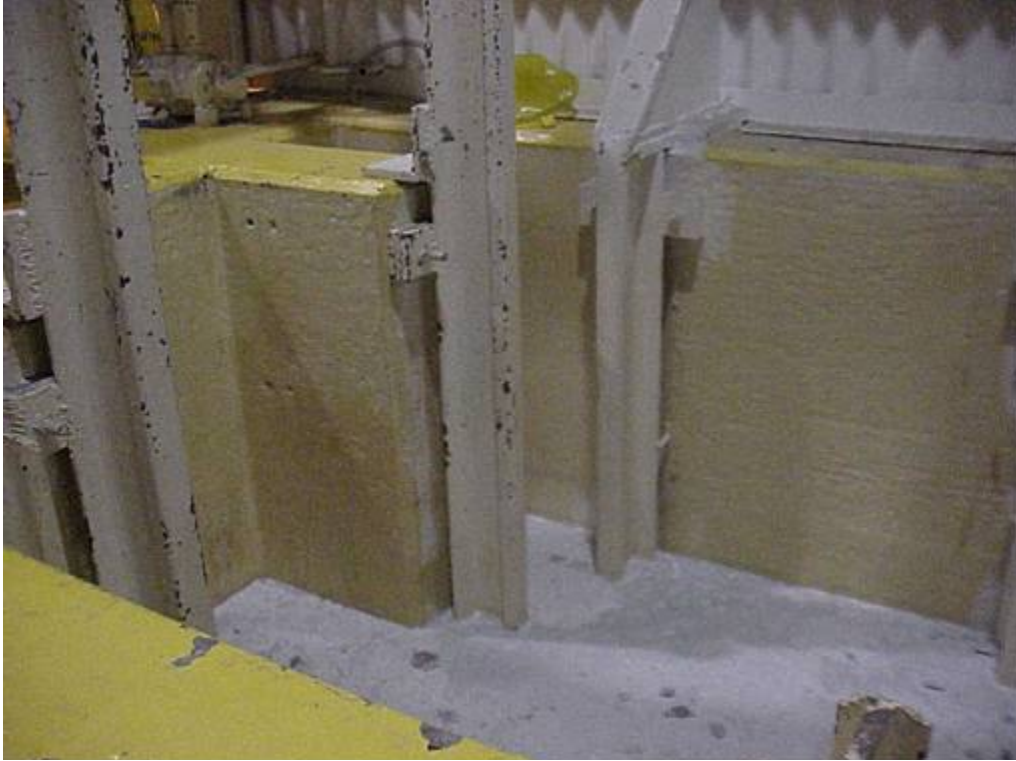
Figure 6. Grouted North Unloading Pit.
