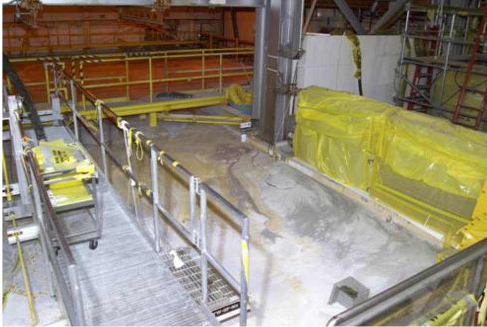
Figure 4. Grouted South Unloading Pit.
