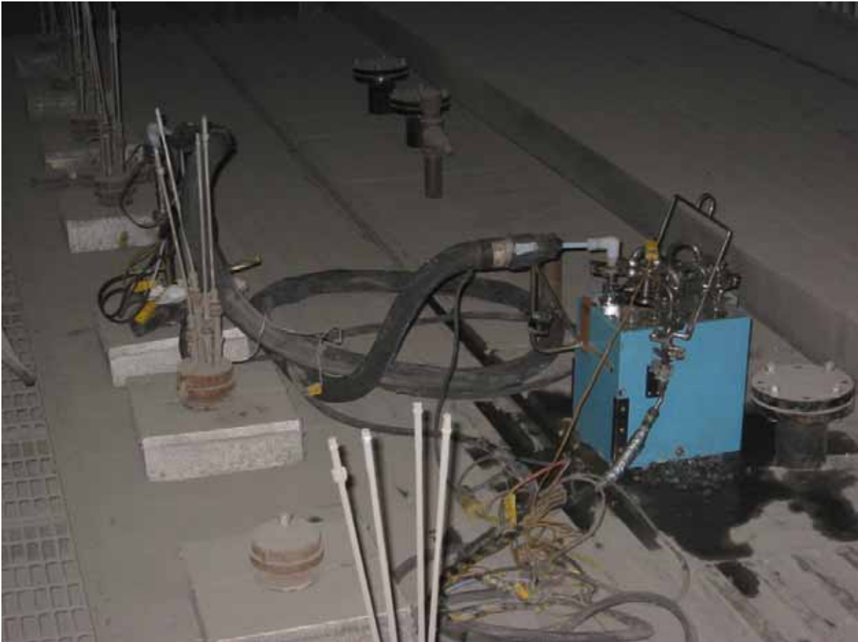
Figure 4. Economizer outlet probe and sampling train
