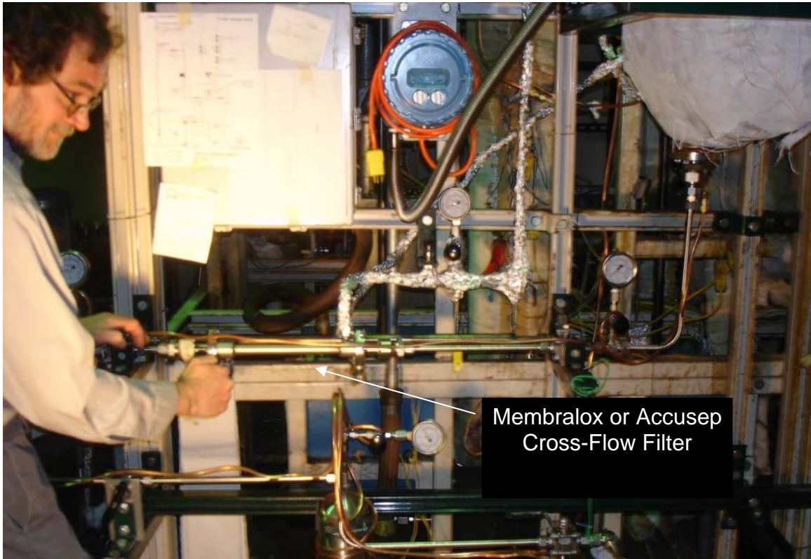
Figure 6. Installation of the Filter Tube Assembly.
