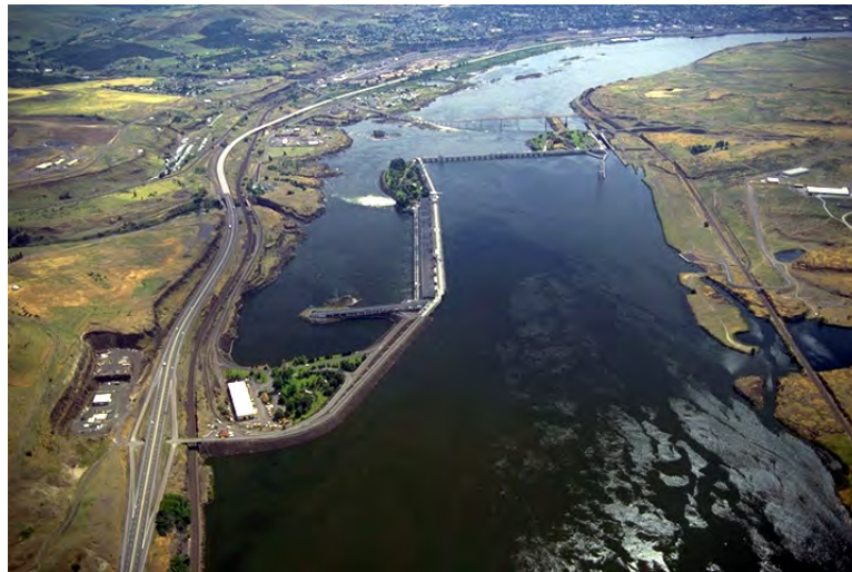
Figure 1.1. Location of The Dalles Project. Looking downstream, the powerhouse is on river left, running parallel to the shoreline; the spillway is across the channel.
