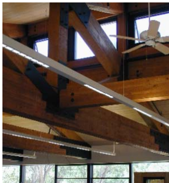
Figure 3-16 Zion's 88% uplighting with T-8 fixtures (note the dark ceilings and beams combined with minimal down lighting)
