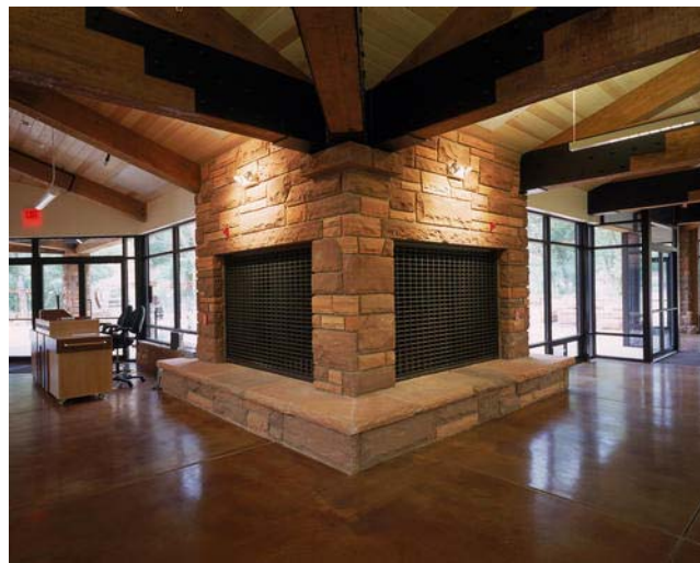
Figure 3-30 Interior view of a cooltower showing operable shutters that allow cool air to enter the building through the bottom louvers
