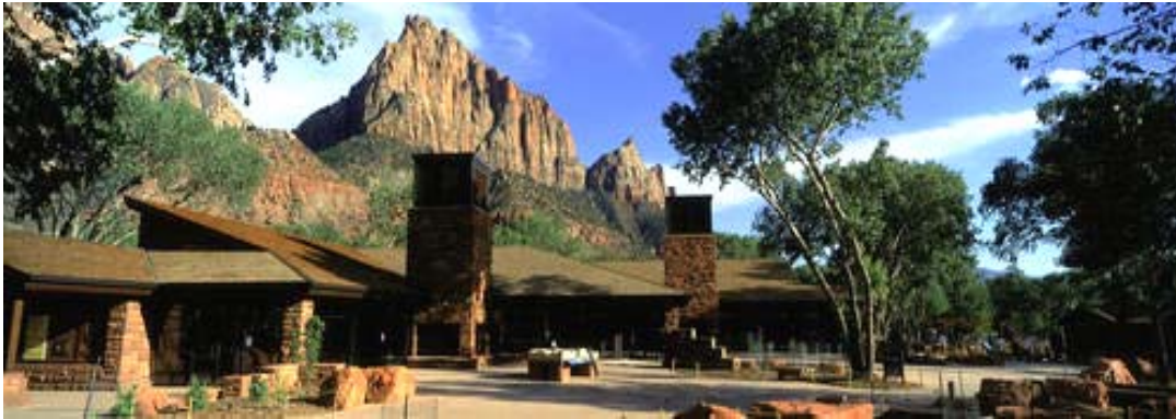
Figure 2-2 North elevation of the Zion Visitor Center showing cooltowers and plaza
