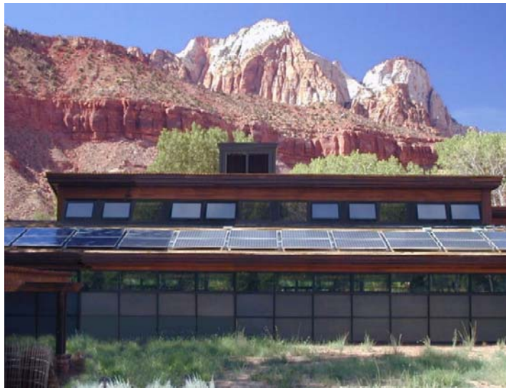
Figure 3-36 Tree shading of Zion PV array
