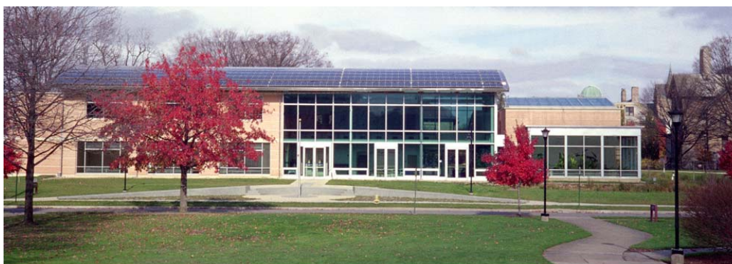
Figure 2-1 South elevation of Oberlin showing roof-mounted PV array
