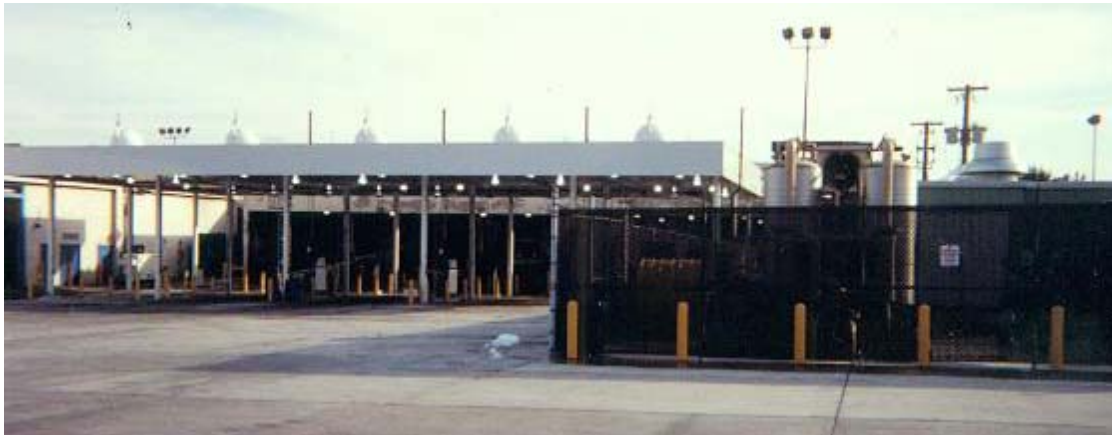
Figure 6. CNG Fueling Area at Bladensburg
