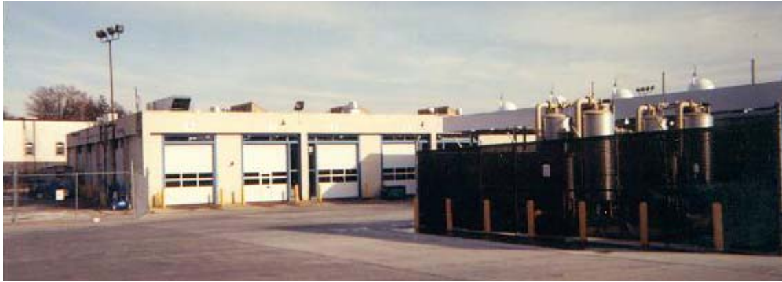
Figure 8. Maintenance Facility at Bladensburg
