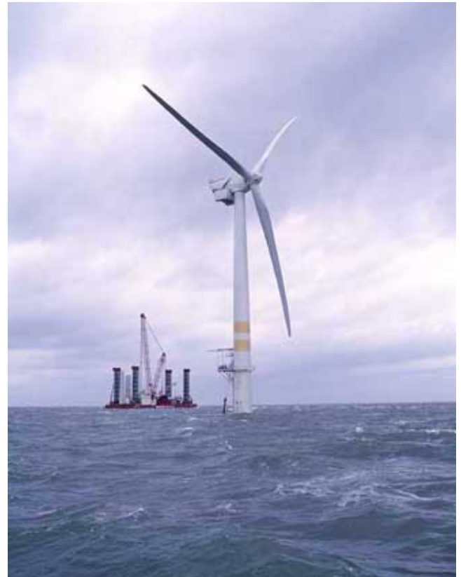
Figure 4 – Typical Offshore Wind Turbine (courtesy of GE)
