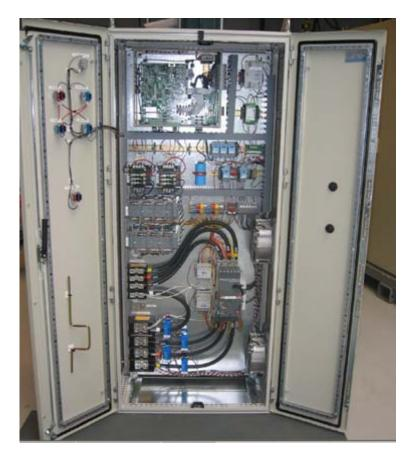
Figure 34. A look inside the DER Switch unit (controller is on upper left)
