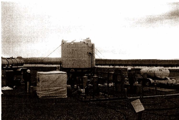
Figure 2. Treatability test equipment, including an above-ground mixing tank, has been installed in the 100 K Area.
