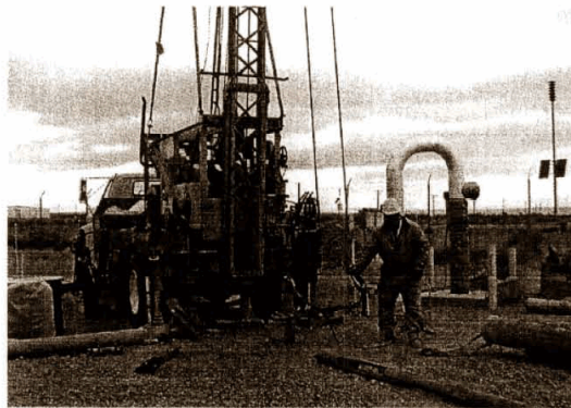
Fig. 4. Wells are drilled on the central Hanford plateau to extract contaminated water.
