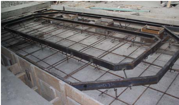
Figure 2: General view of the NESTOR ring foundation.
