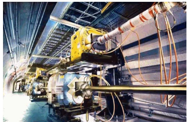
Figure 2. Tunnel view of PEP-II
