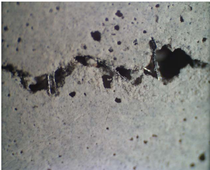
Figure 7 – Bridging of concrete composite fracture by CMS fibers
