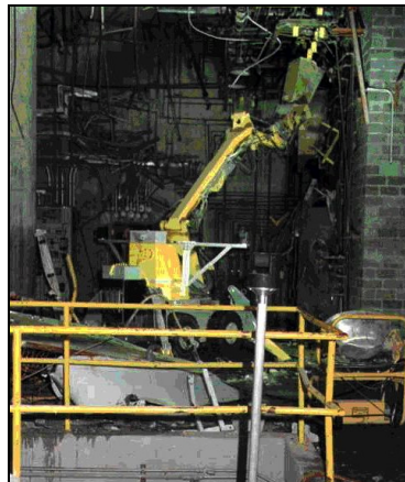
Fig. 10. Modified Brokk performing facility D&D task.
