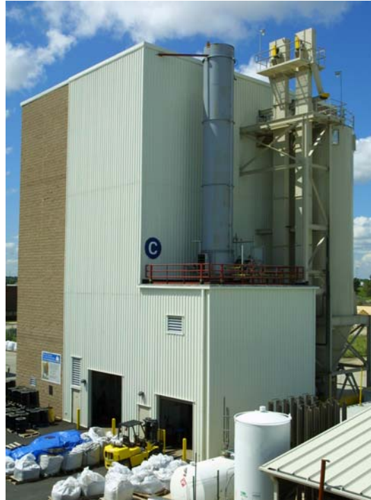
Figure 7 – GTI's Newly-Commissioned Flex-Fuel Test Facility
