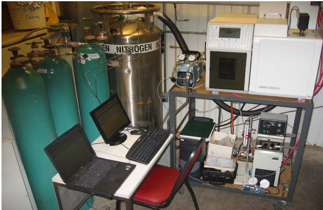
Figure 28 – Trace Sulfur Analysis GC/PPFD Installed at the FFTF Fourth Floor Analytical Station
