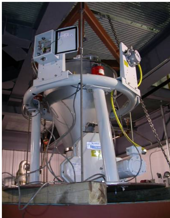
Figure 15 – Loss-in-Weight Fine Sorbent Feeder
