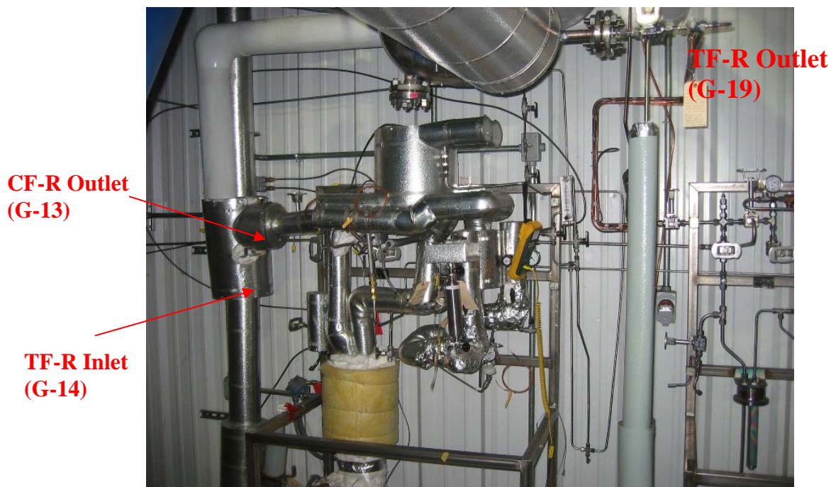
Figure 22 - Photograph of the SE&C Skid #2 at the G-13/G-14 Locations (After Insulation)
