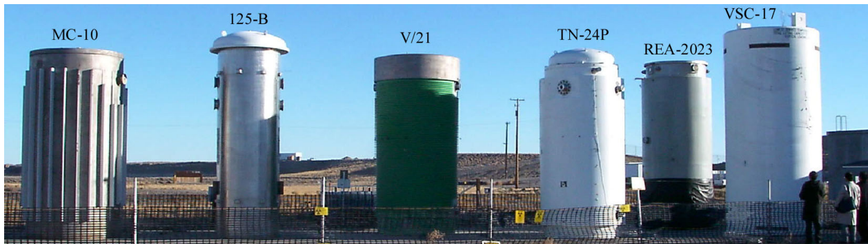
Fig. 1. The six casks available for measurement at the INL Test Area North Facility.
