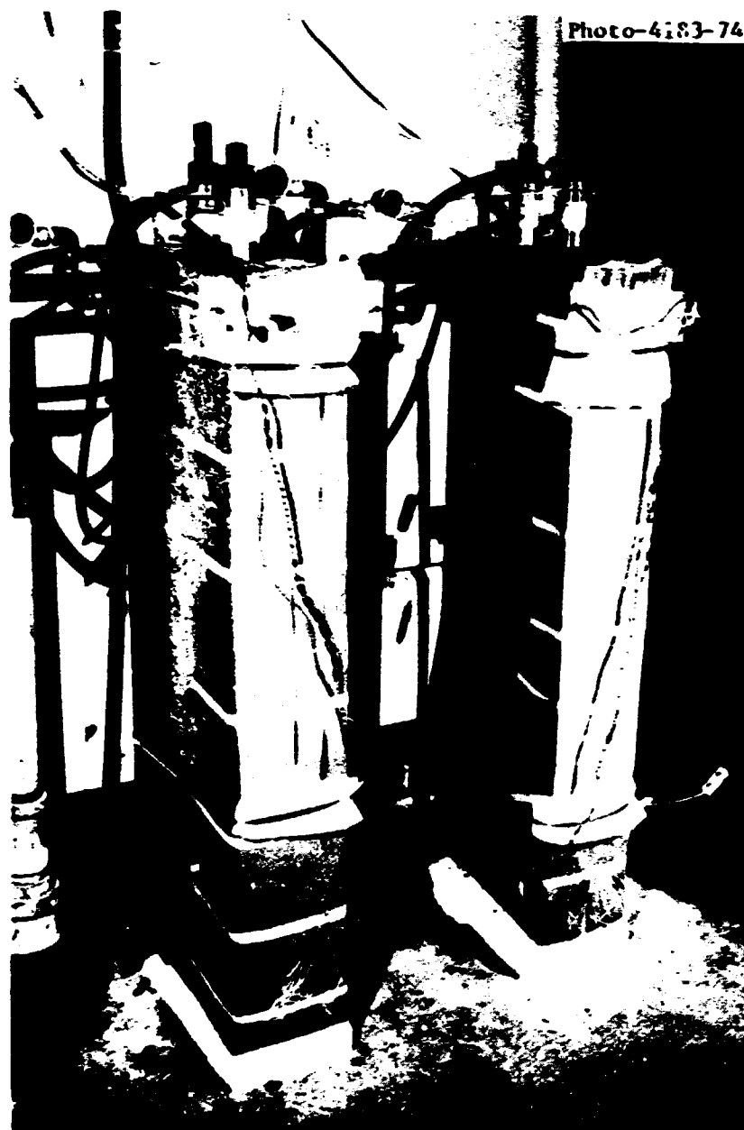
Fig. 6. Panelcoils and Electric Strip Heaters on Segments of Thermal Cylinder Test Before Being Insulated.
