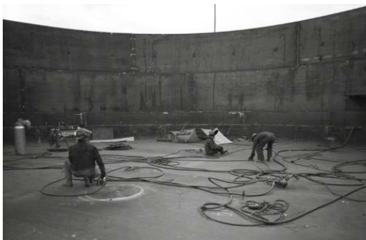
Fabrication of Primary Bottom
