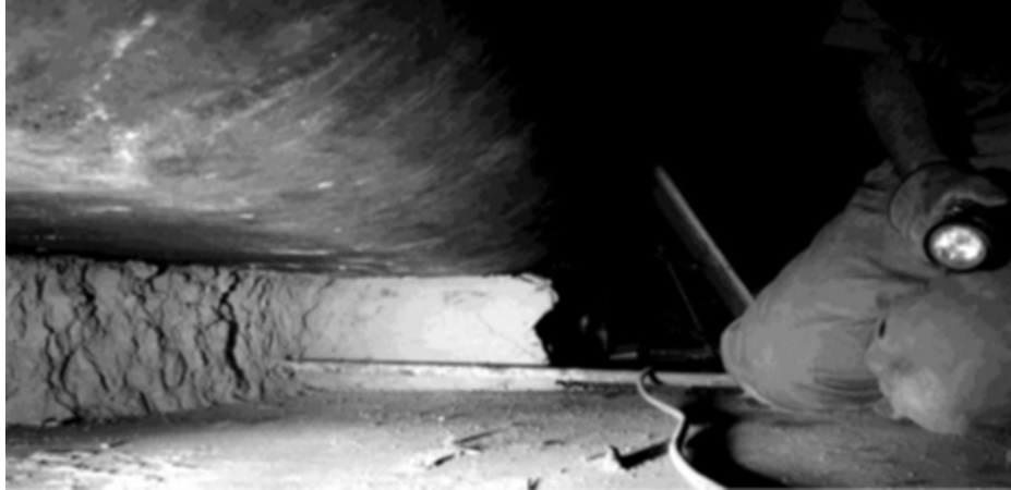
Figure 5. Refractory repair under bottom knuckle of tank AY-102.
