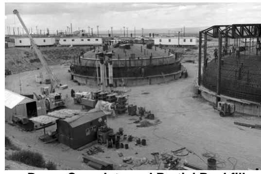
Dome Complete and Partial Backfill
