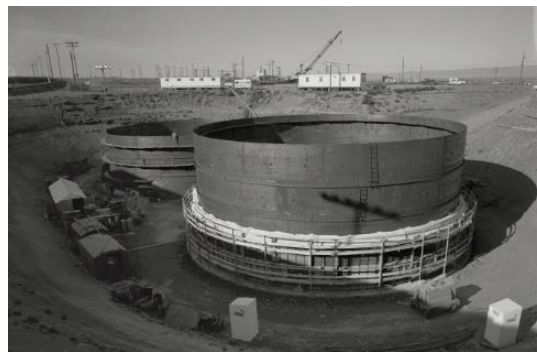
Erection of Secondary Liner and Concrete Wall
