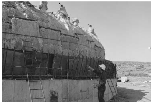
Insulation Prior to Heat Treatment
