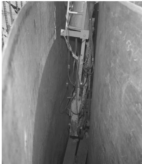
Fig. 3. Challenges in access when welding 241-AY tank farm primary liners.
