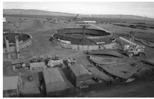
Erection of Dome Plates
