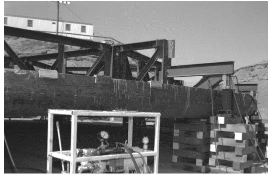
Fabrication of the Secondary Bottom
