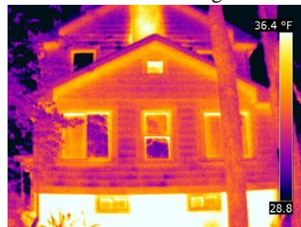
Fig. 49. Infrared image of west end of Gaiter house.
