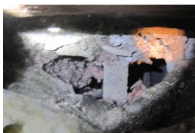
Fig. 69. Opening to interior walls in attic.
