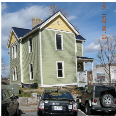
Fig. 36. Green House, during the rehabilitation process, with restored exterior.
