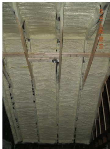
Fig. 23. Attic was first sprayed with 1 in. of closed-cell foam.
