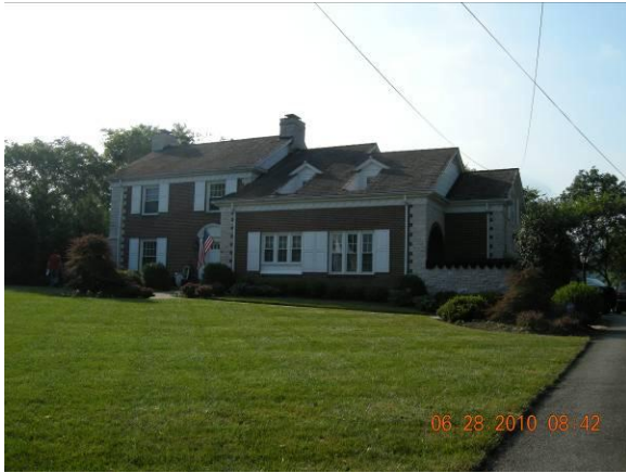
Fig. 64. Eagle Bend, in Clinton, Tennessee.
