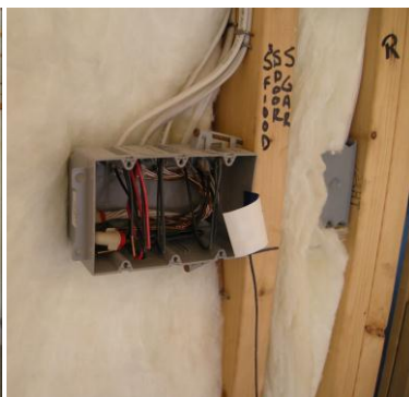
Fig. 10. Wall between garage and kitchen and close-up of electrical box. (Notice electrical switch boxes form a potential short leakage path.)
