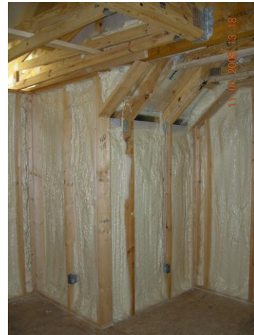
Fig. 5. Foam sealed knee walls. Source: Jeff Christian et al., Tennessee Valley Authority’s Campbell Creek Energy Efficient Homes Project: 2010 First Year Performance Report July 1, 2009–August 31, 2010 , Fig. 86.
