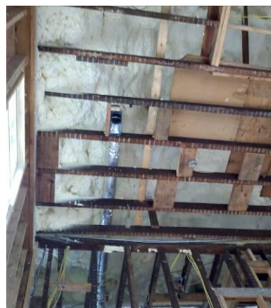
Fig. 38. Spray foam applied to underside of roof.
