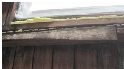
Fig. 47. Low-expansion foam around window.
