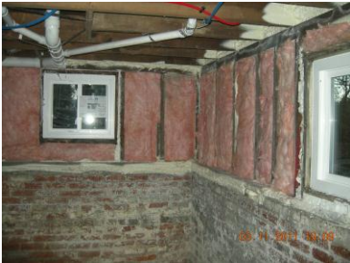
Fig. 16. Rim joist (at top of picture) is well-insulated and sealed.
