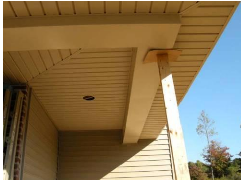
Fig. 29. Front porch box beam.
