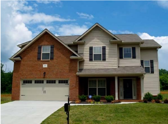
Fig. 26. Campbell Creek retrofit house, CC2.
