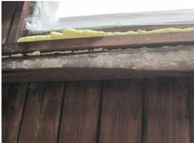
Fig. 17. Foam insulation around windows.
