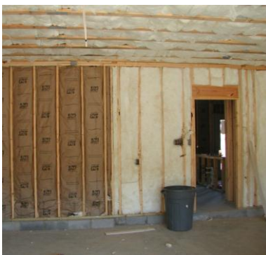
Fig. 10. Wall between garage and kitchen and close-up of electrical box. (Notice electrical switch boxes form a potential short leakage path.)
