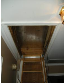
Fig. 7. Insulated and sealed attic opening.
