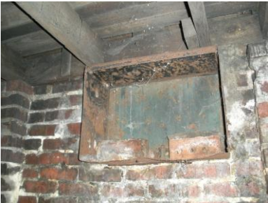
Fig. 15. Uninsulated rim joists.
