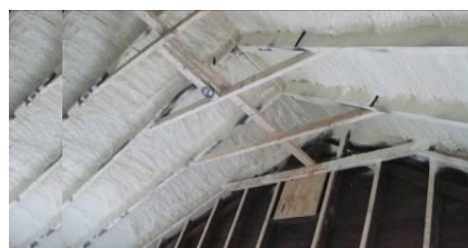
Fig. 46. SPF shortly after application to underside of roof.
