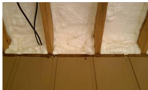
Fig. 35. Sprayed foam insulation in porch roof.
