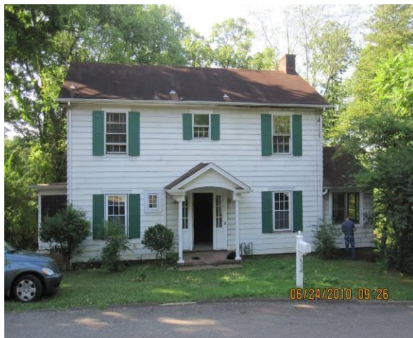
Fig. 45. Historic Gaiter house was gutted before renovation.
