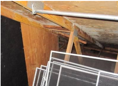
Fig. 75. Open chase into home from attic.
