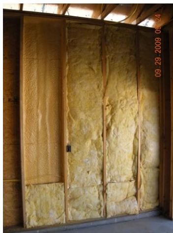
Fig. 22. Flash-and-batt insulation.
