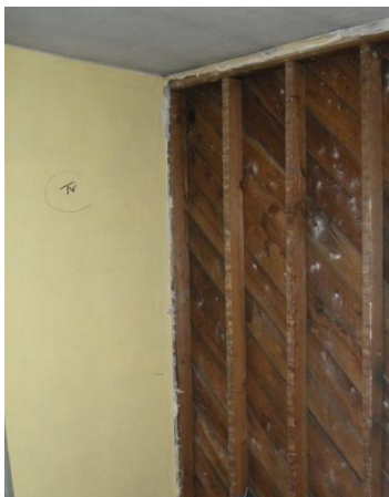
Pre-retrofit walls with no insulation
