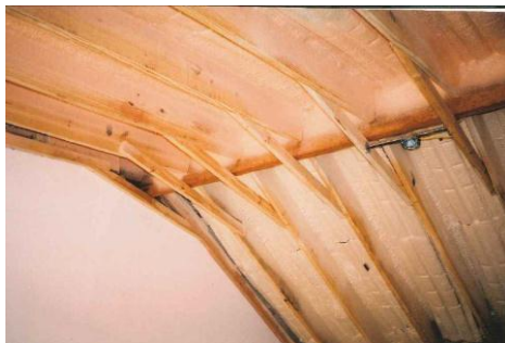
Spray foam insulation on the living room cathedral ceiling (left photo) and the kitchen walls (right photo).
