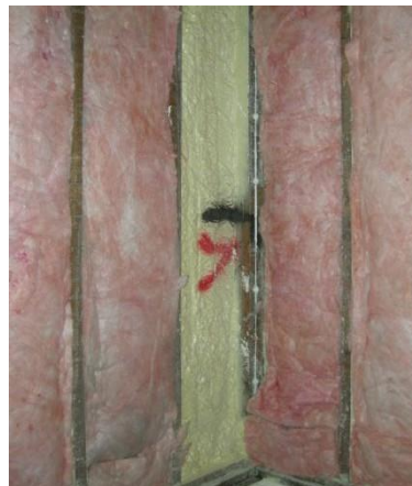
Post-retrofit wall with flash and batt
