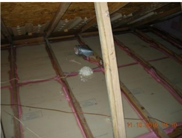
Pink Latex foam used to seal the attic floor.
