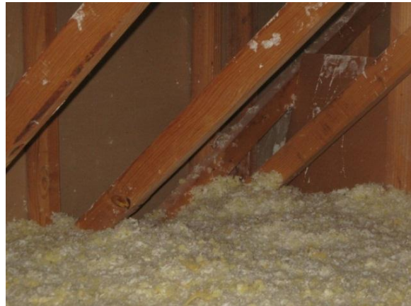
Fig. 8. Attic insulation upgraded to R-38.
