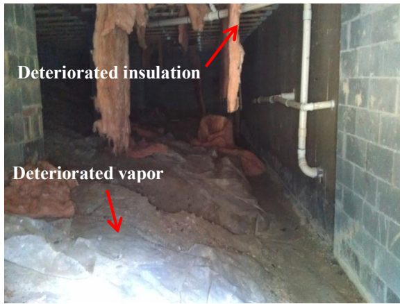
Fig. 9. Existing insulation and vapor barrier in the crawlspace.
