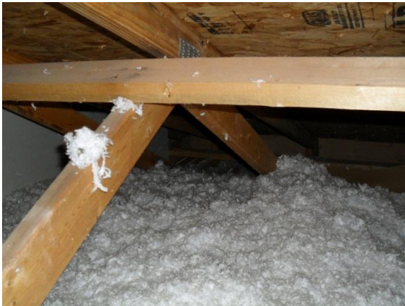
Fig. 7. Existing R-30 insulation in the attic.
