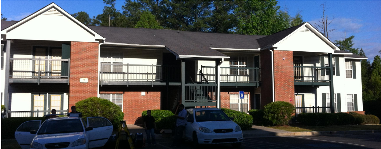
Fig. 2. View of Building #7 in Mapewood Park Apartments.
