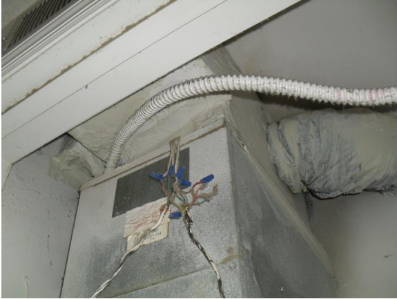
Fig. 11. Existing indoor unit the air handler.
