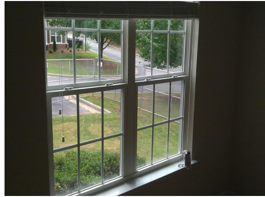
Fig. 6. New double-pane, low-e, vinyl-frame windows.
