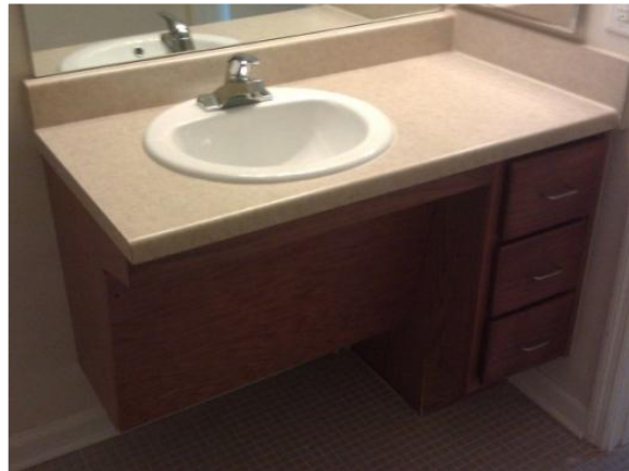
Fig. 16. New plumbing fixtures
