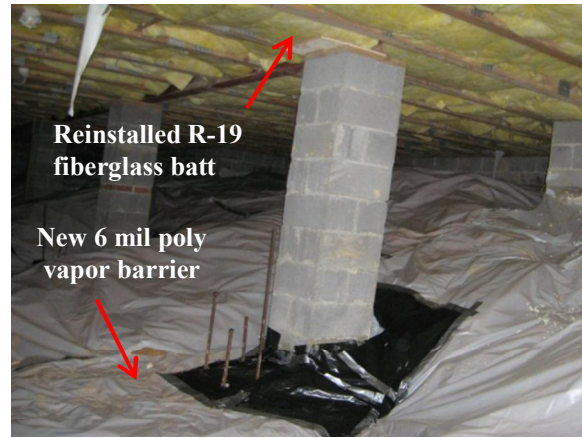
Fig. 10. New insulation and vapor barrier in the crawlspace
