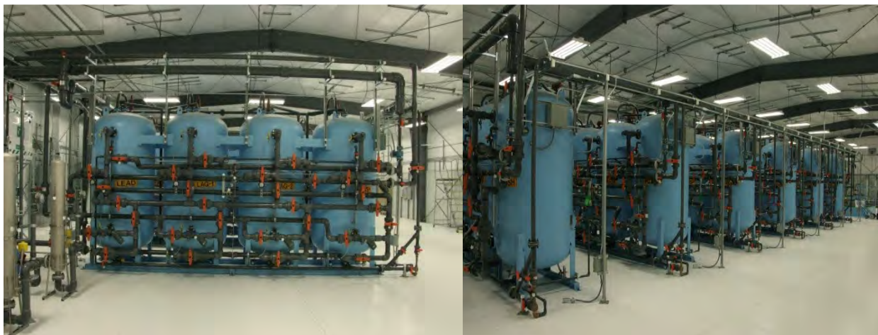
Fig. 3. Ion Exchange trains at DX pump-and-treat
