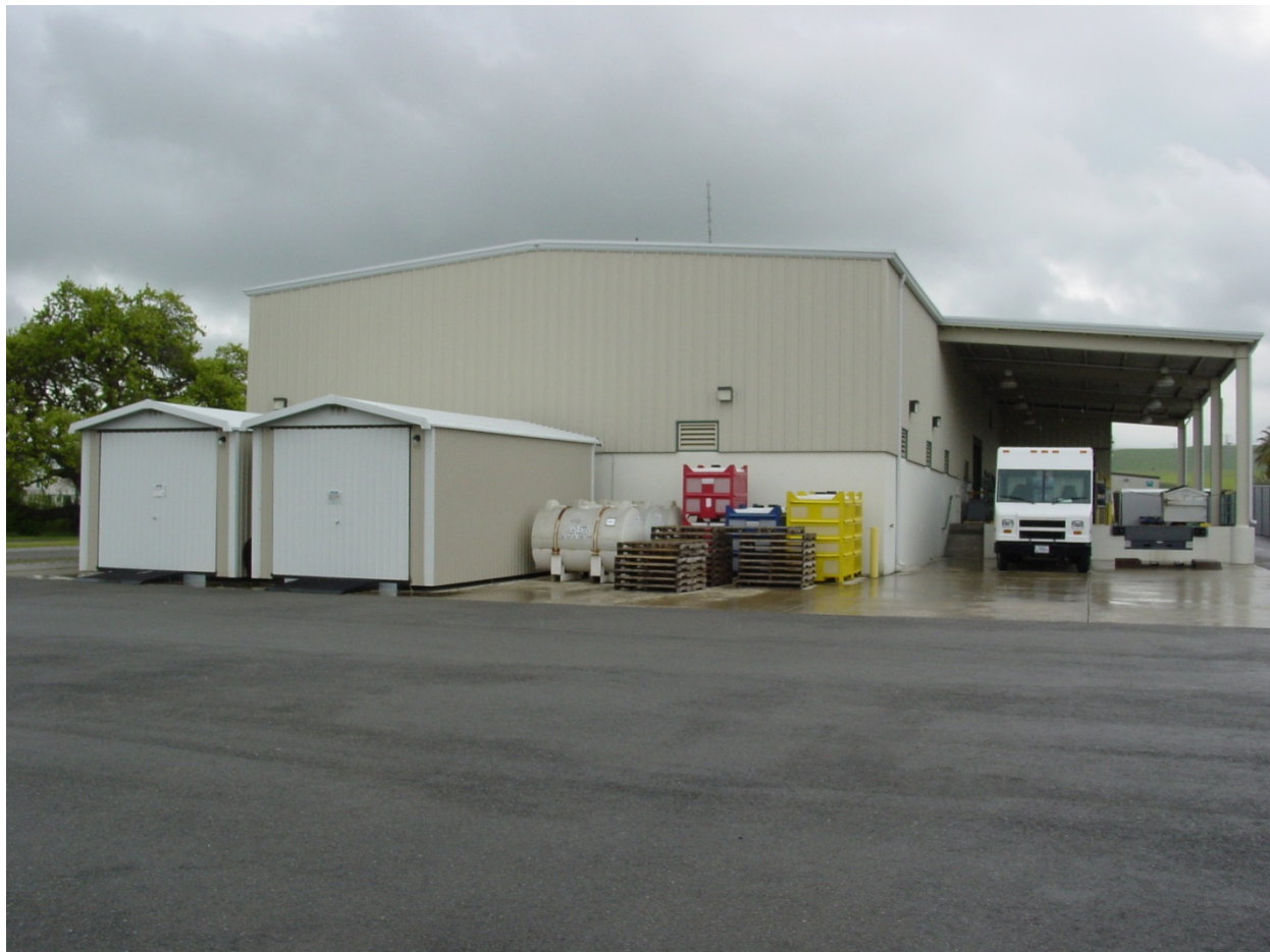
Figure 1-2 Waste Management Facility Building 9611
