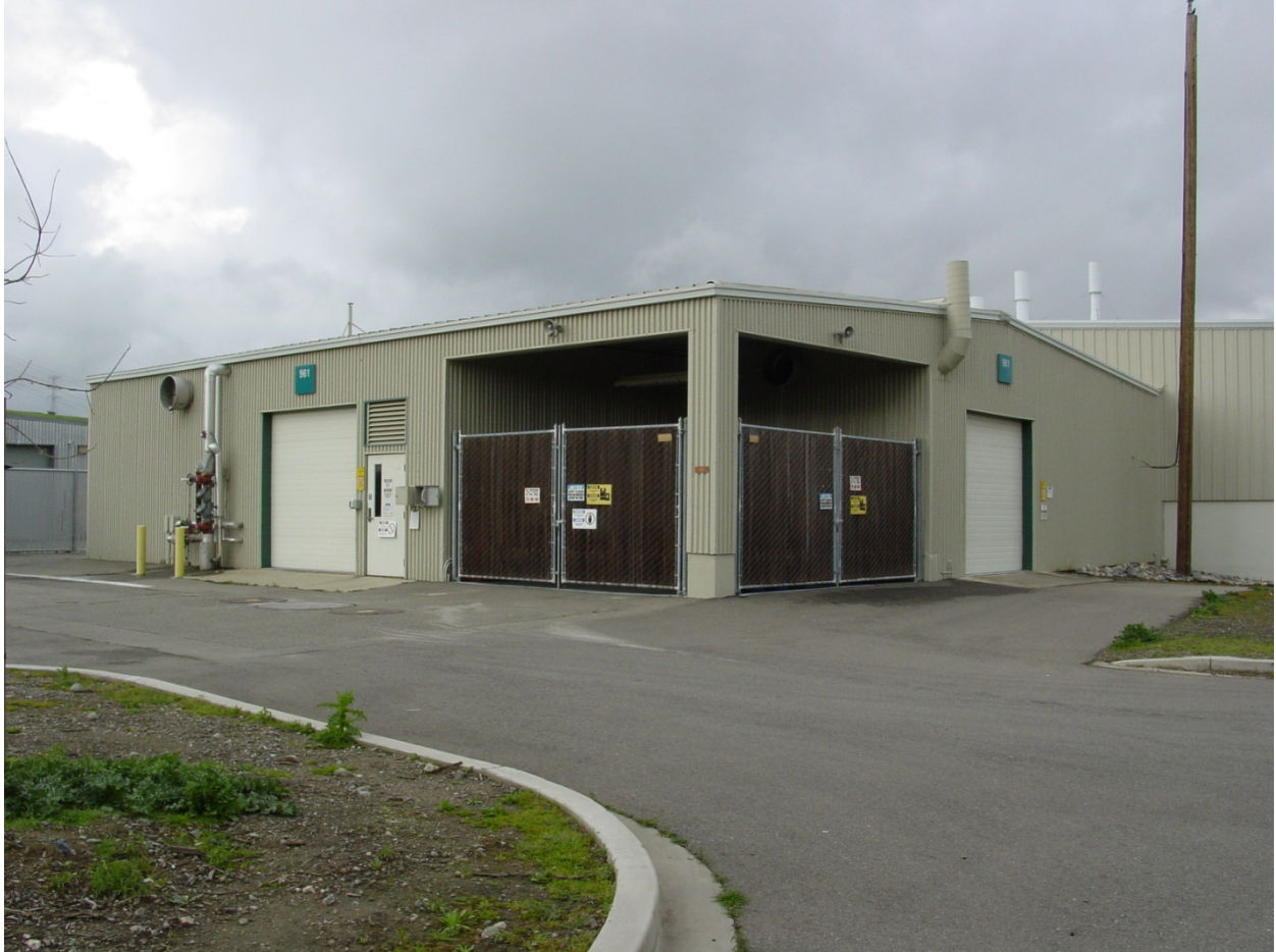
Figure 1-1 Waste Management Facility Building 961
