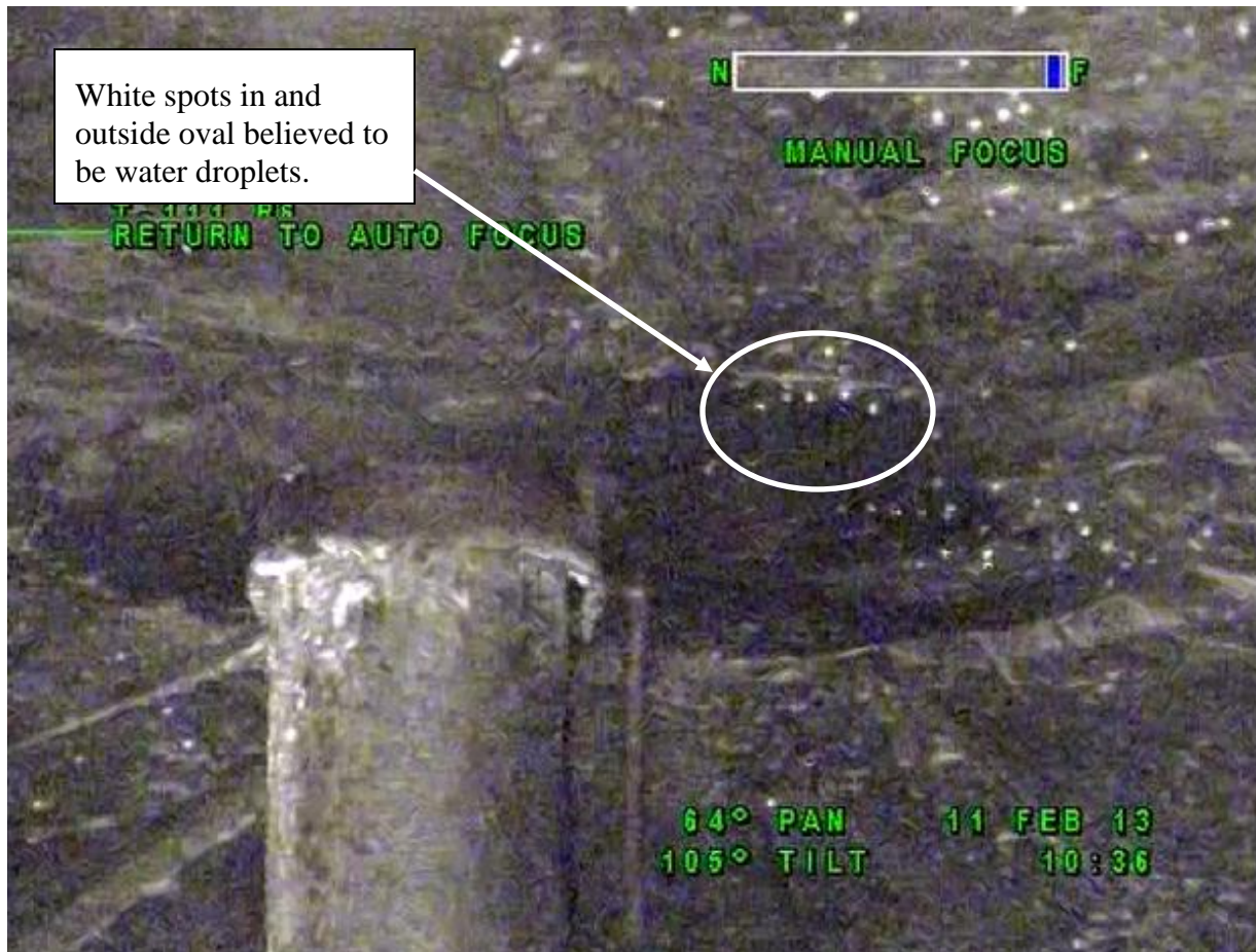
Figure 11 Tank T-111 Central Dome Area Showing Probable Water Droplets
