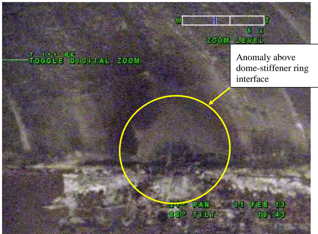
Figure 9 Anomaly on SE Area of Tank T-111 Dome Just Above Top Stiffener Ring
