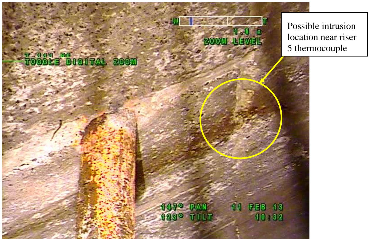
Figure 7 Possible Past Intrusion Location in Tank T-111 Dome
