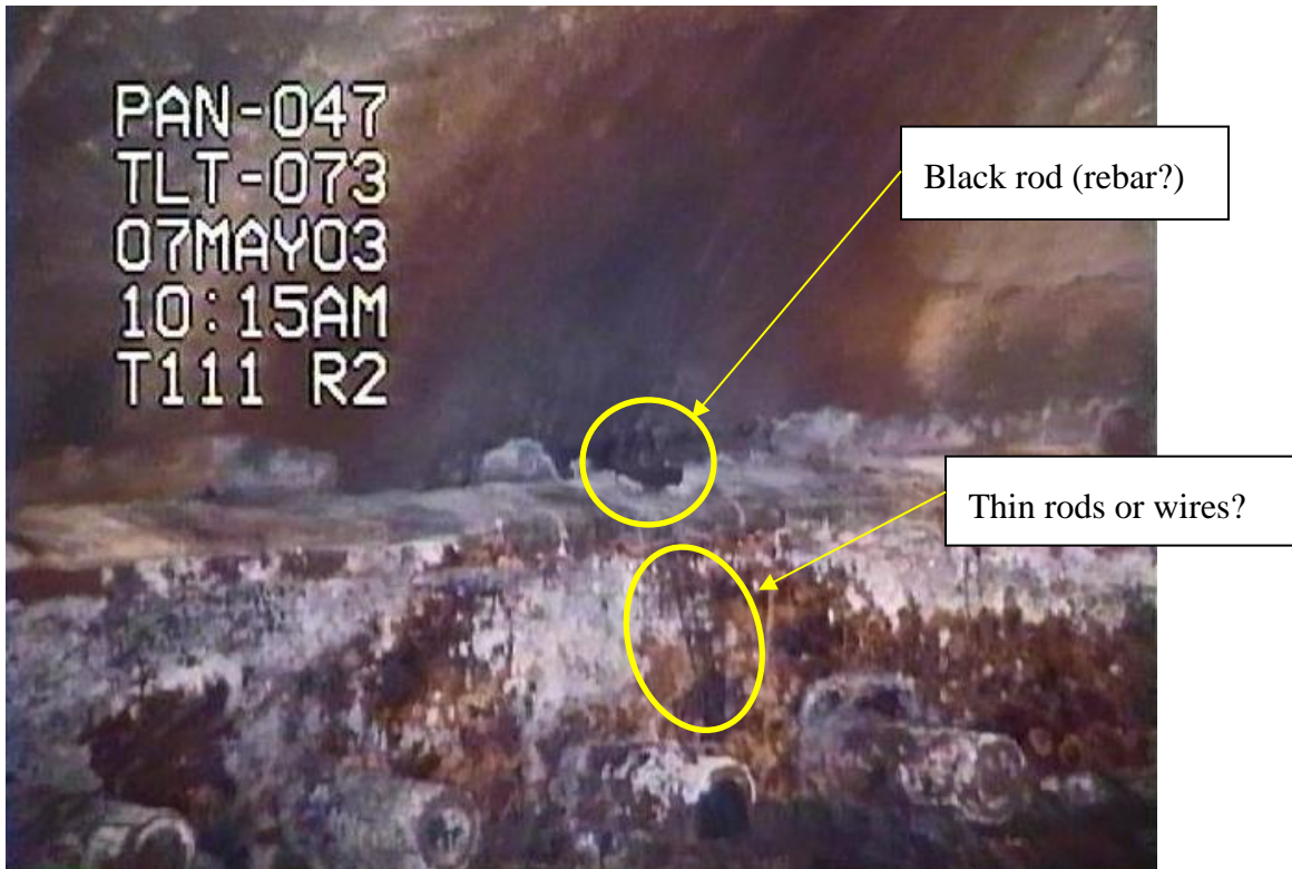
Figure 5 Anomaly on East Wall of Tank T-111 on May 7, 2003
