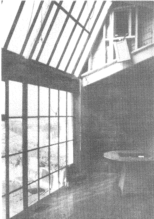
Diffuse north light is a widely recognized tradition for artists' studios. Studio space in the San Francisco Art Institute typically utilizes large north-facing glazed areas.
