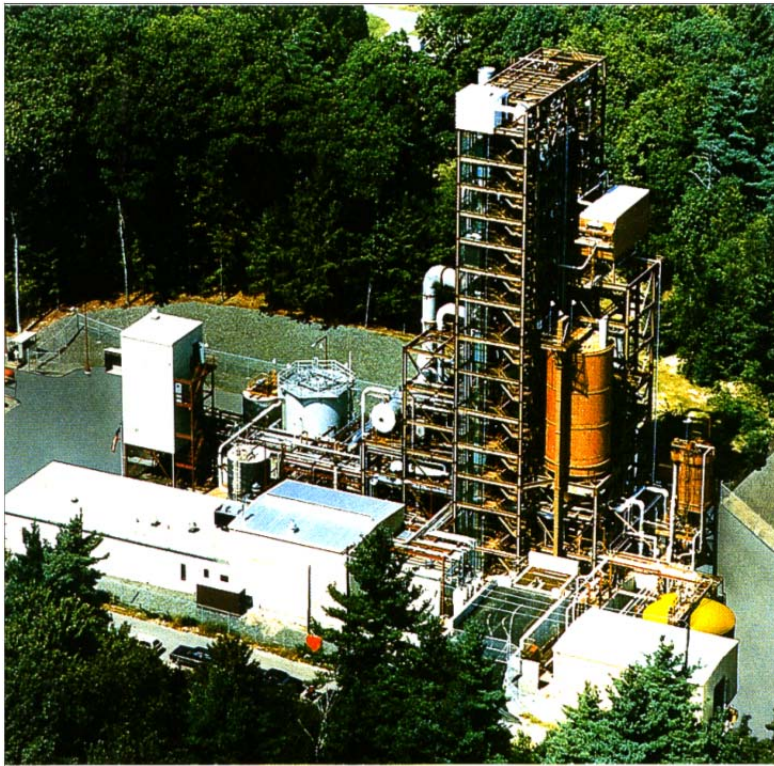
Figure 3-1 - The Windsor Connecticut Coal Gasification Pilot Plant.
