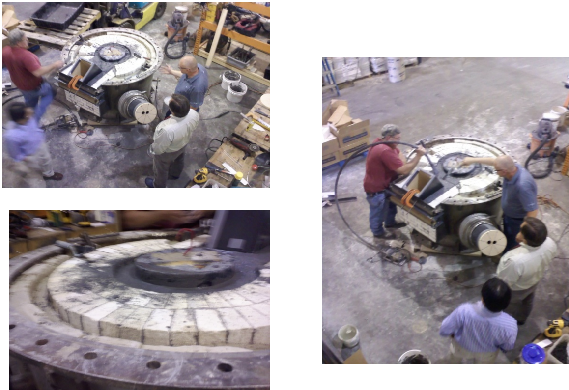
Figure 5-9 – Lower Oxidizer refractory installation by LVR
