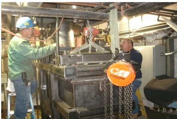
Figure 5-14a (left) – USPCV being installed Figure 5-14b (right) – Reducer Bottom Outlet
