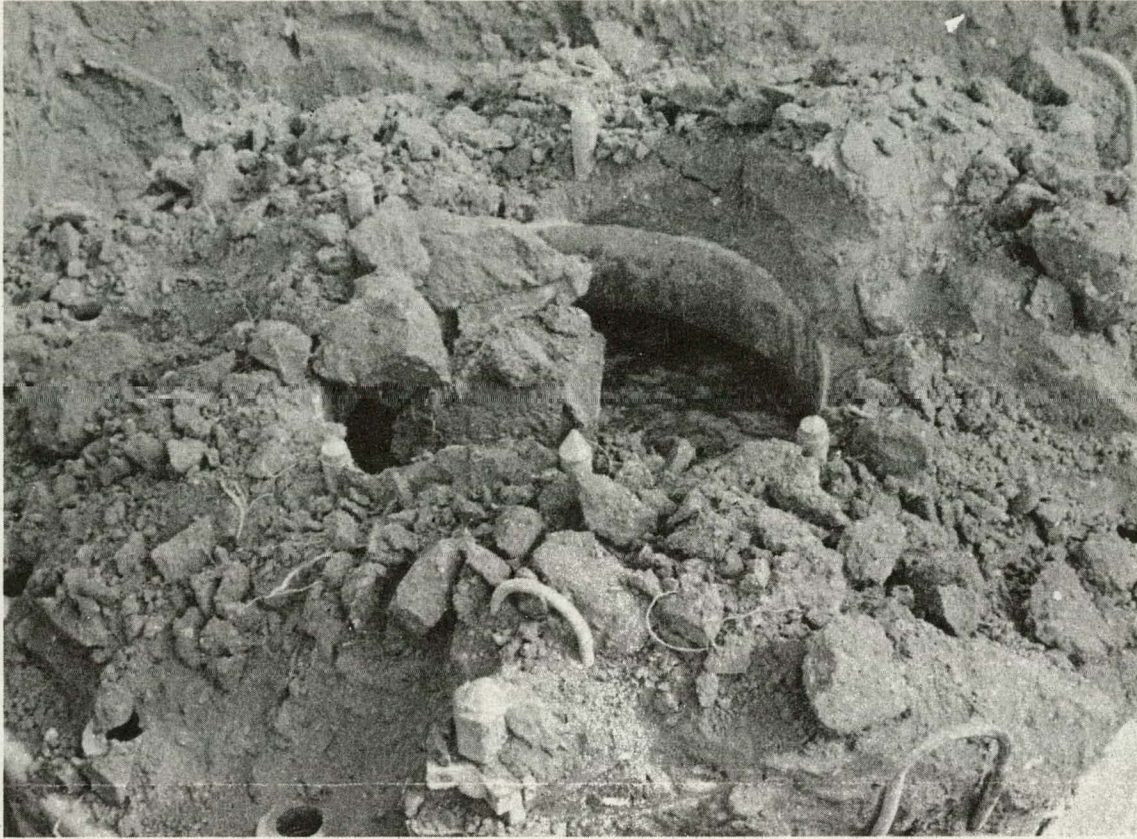
FIGURE 5. Buried Purex Feed Adjustment Tank Filled With Soil and Water
