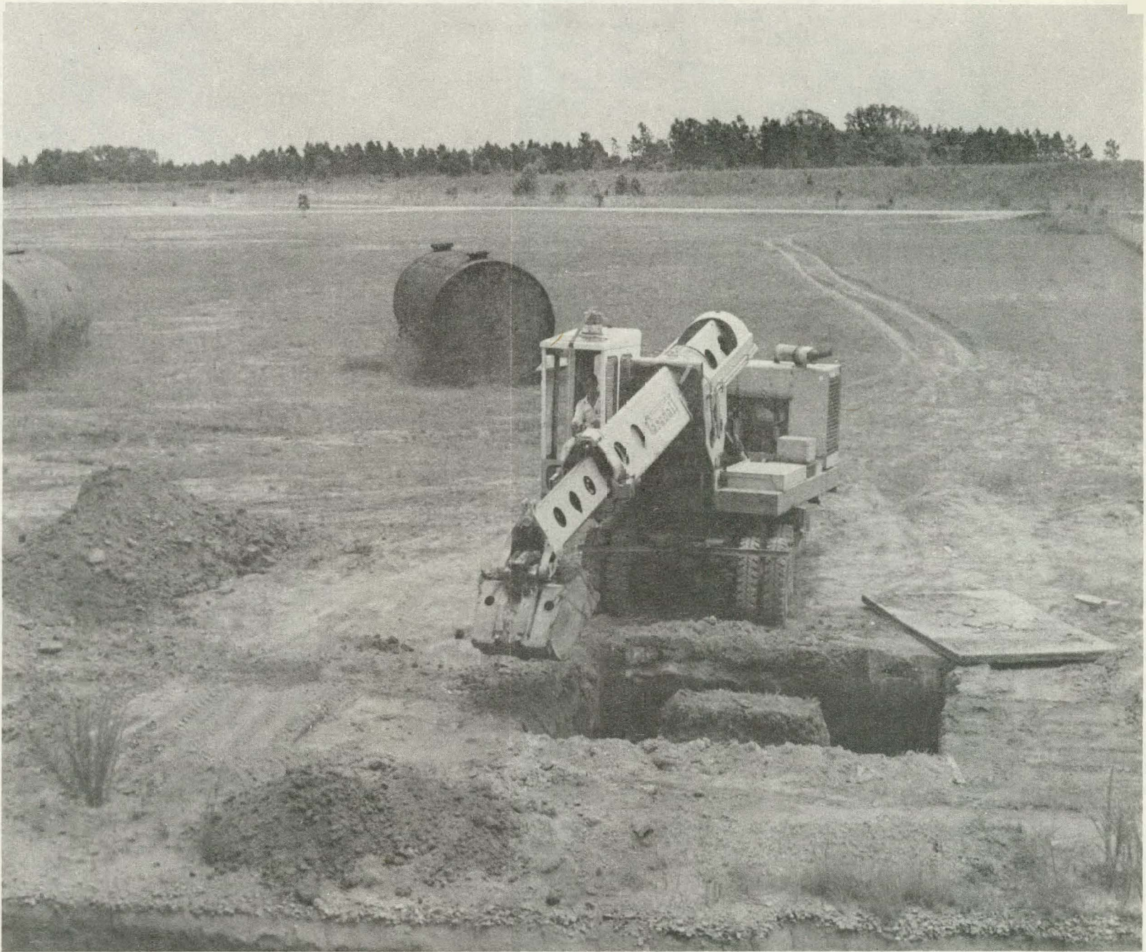
FIGURE 14. Excavation of Lysimeter Pit
