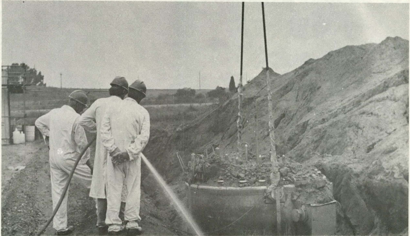
FIGURE 7. Washing Exterior of Exhumed Purex Feed Adjustment Tank
