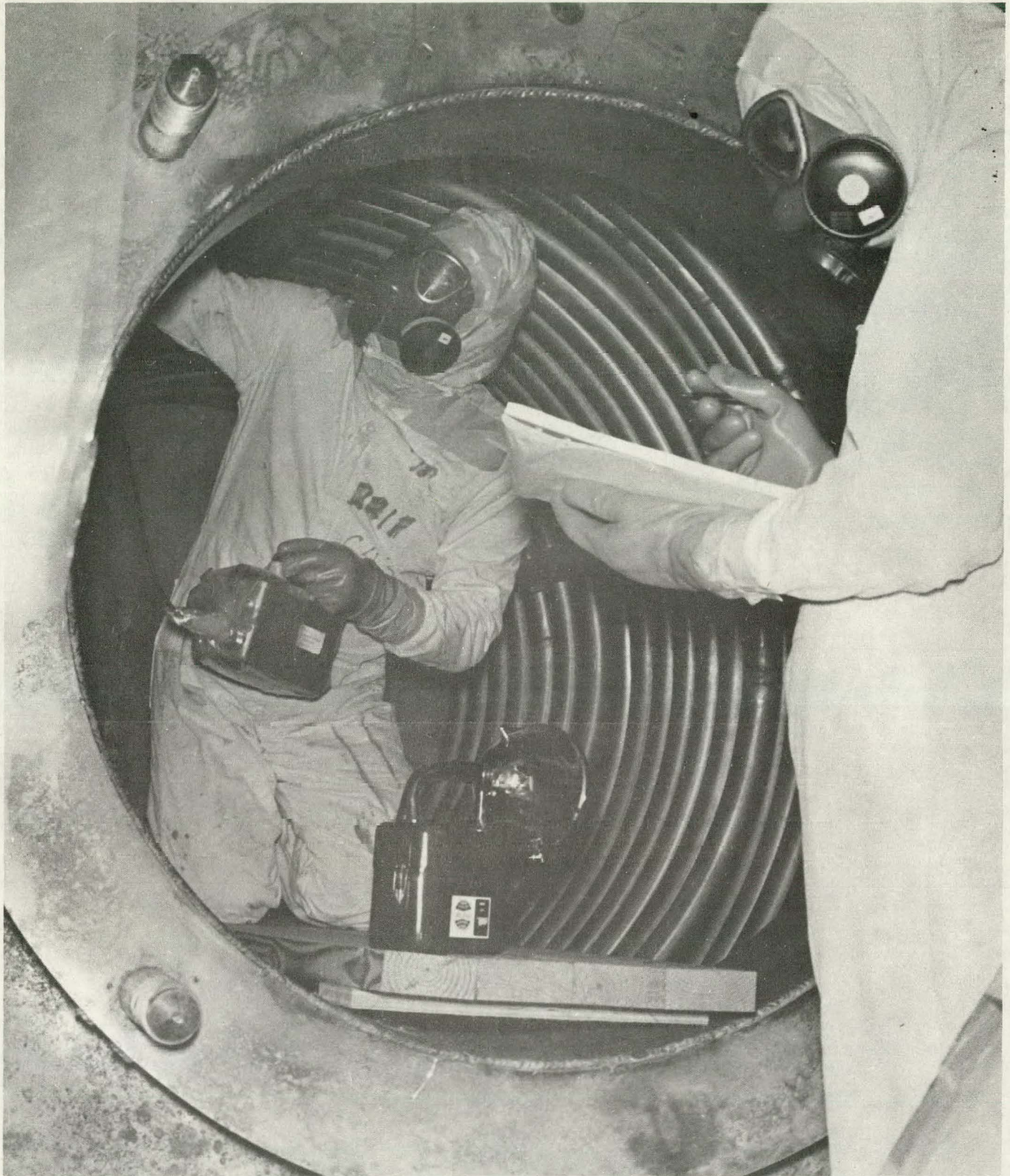
FIGURE 11. Alpha Activity Survey of Interior of Exhumed Purex Feed Adjustment Tank After Mud Removal
