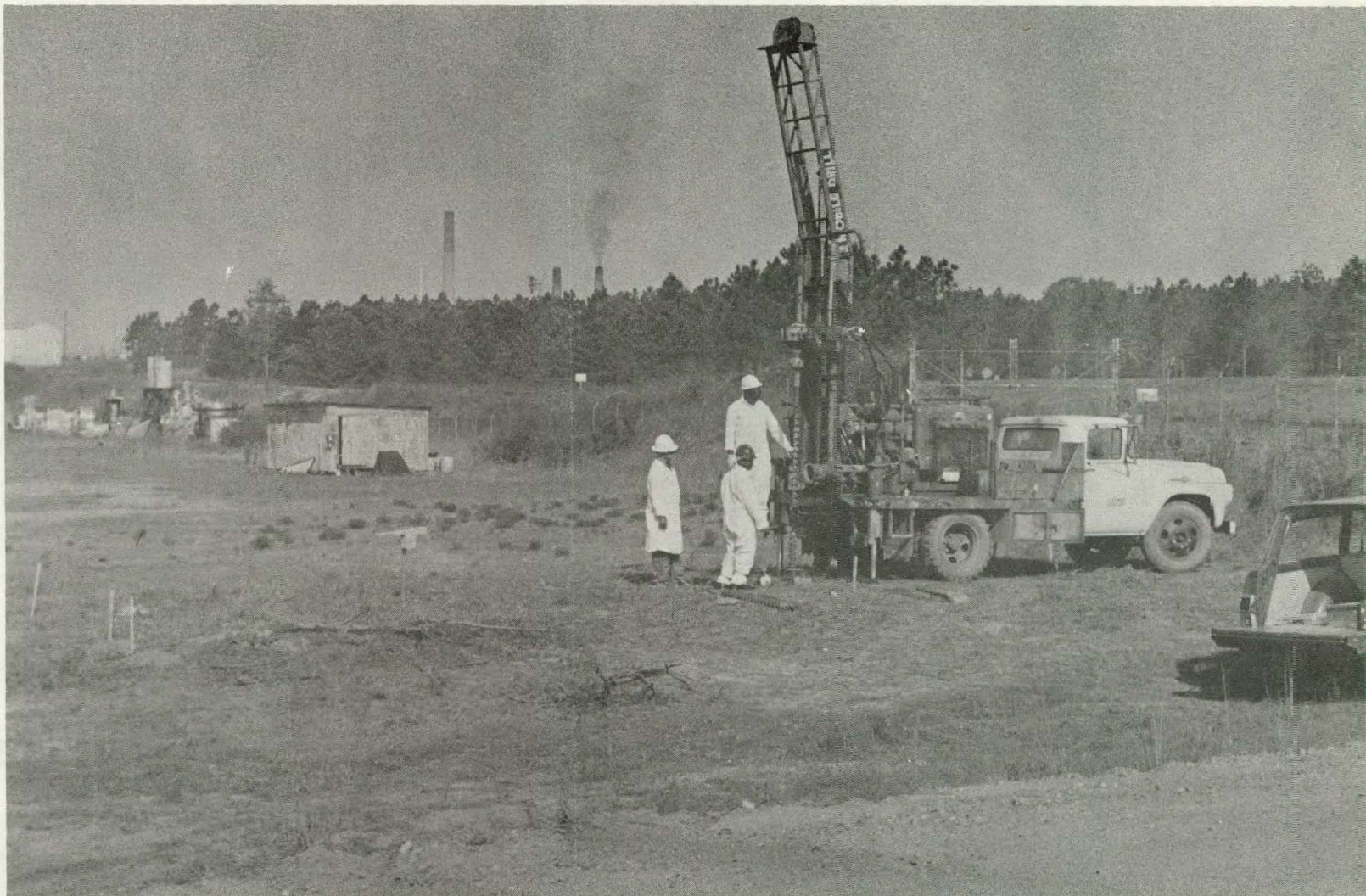
FIGURE 1. Drill Probing for Buried Process Vessel
