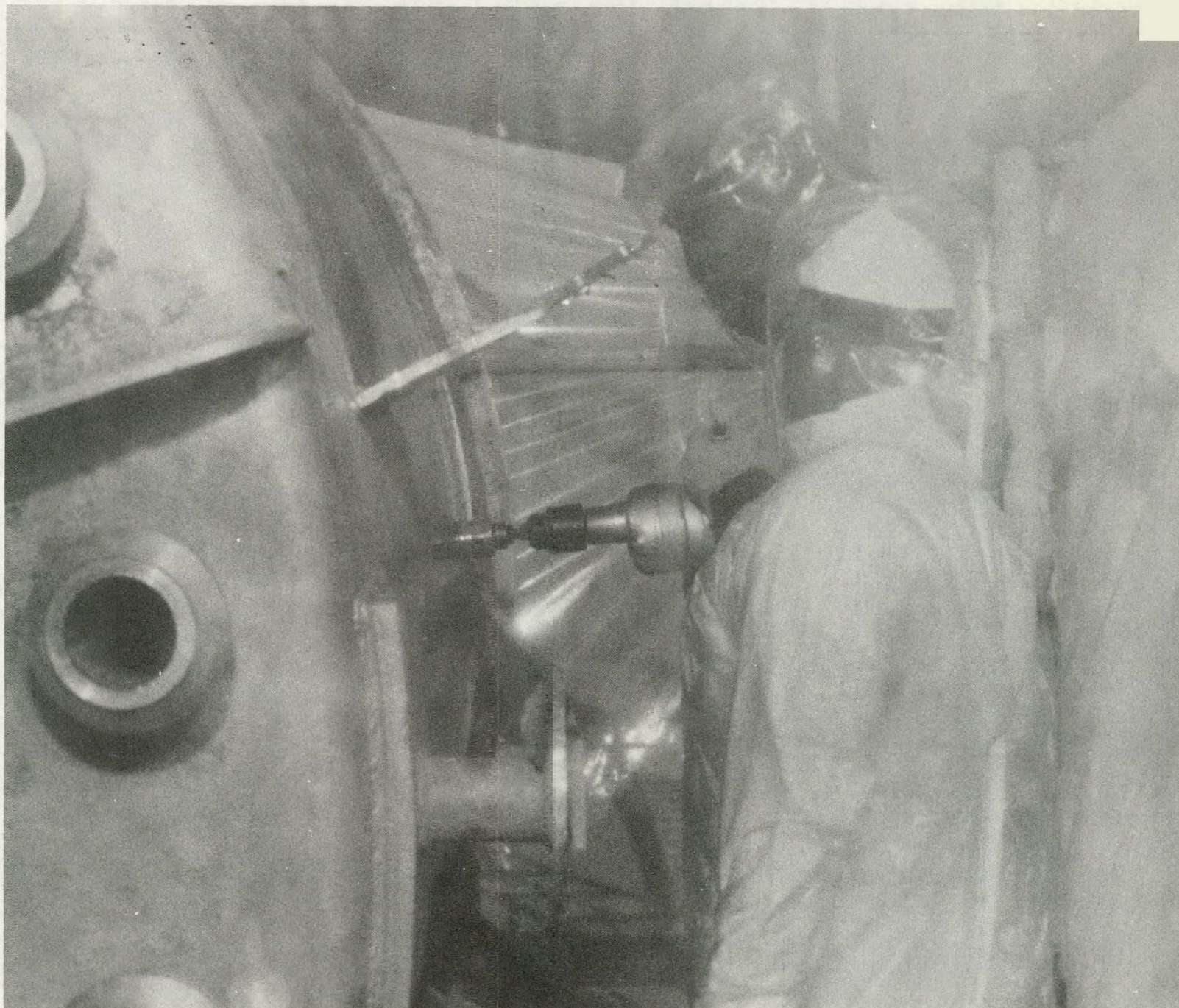
FIGURE 13. Cutting Sample Coupons from Exhumed Purex Feed Adjustment Tank
