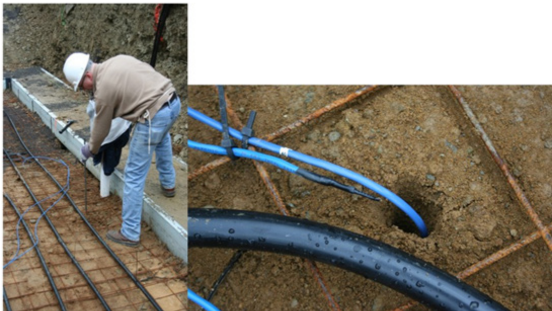
Figure 6. Typical soil TC installation
