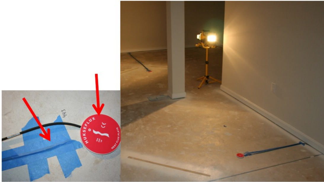
Figure 9. Typical installation of basement floor TC and heat flux sensor
