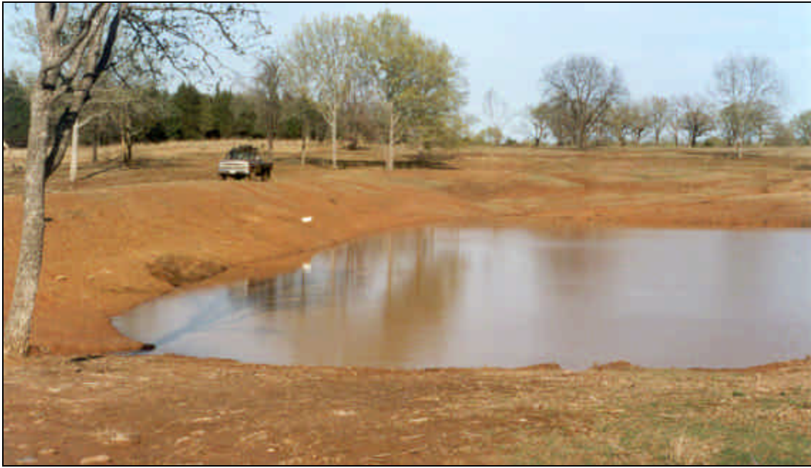
Figure 4. Dam 1 (spillway in background).
