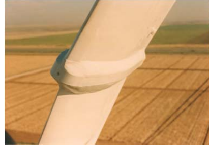
Figure 18. Fairing over Blade-to-Blade Joint.
