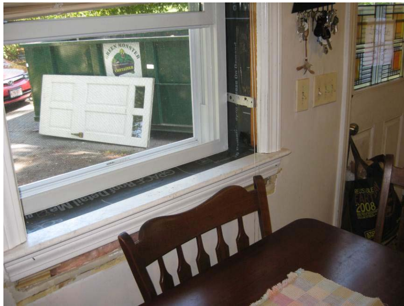
Figure 11. Millbury Cape “outie” windows
