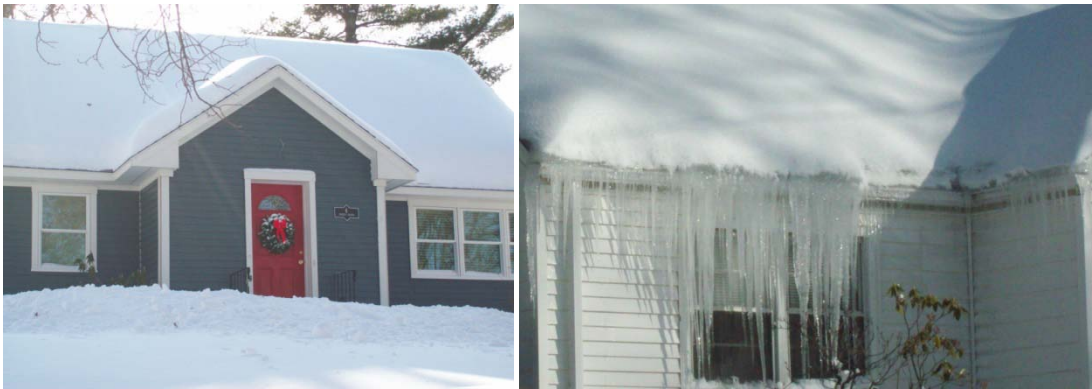
Figure 25. Left: Post-retrofit Millbury Cape; Right: Neighbor’s home with ice dams
