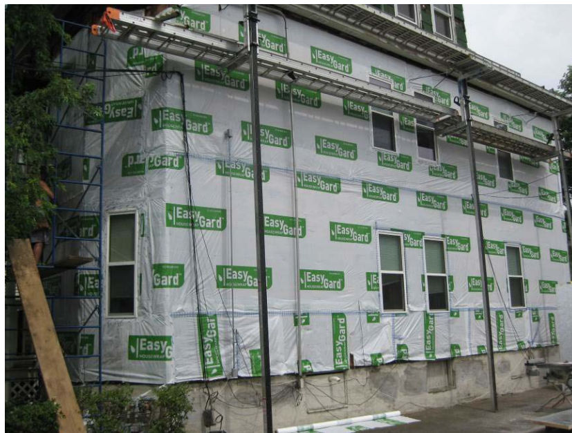
Figure 13. Somerville Triple Decker exterior wall air barrier
