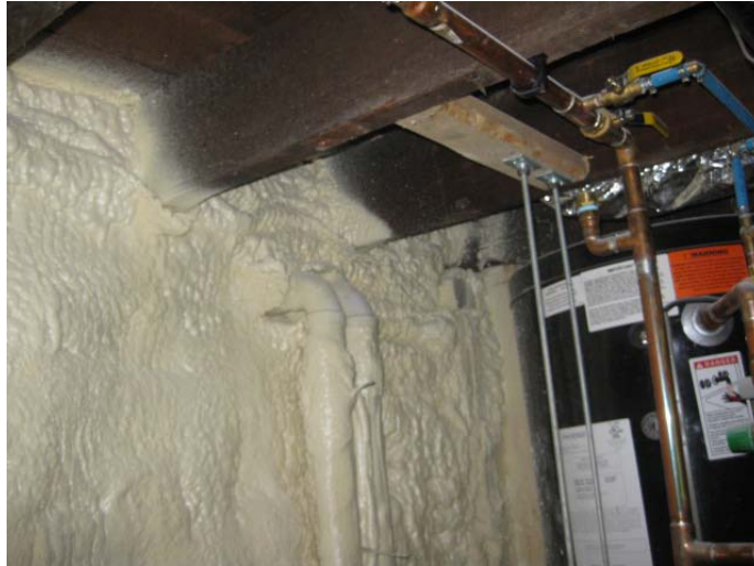
Figure 8. Somerville Triple Decker basement wall insulation before application of ignition barrier
