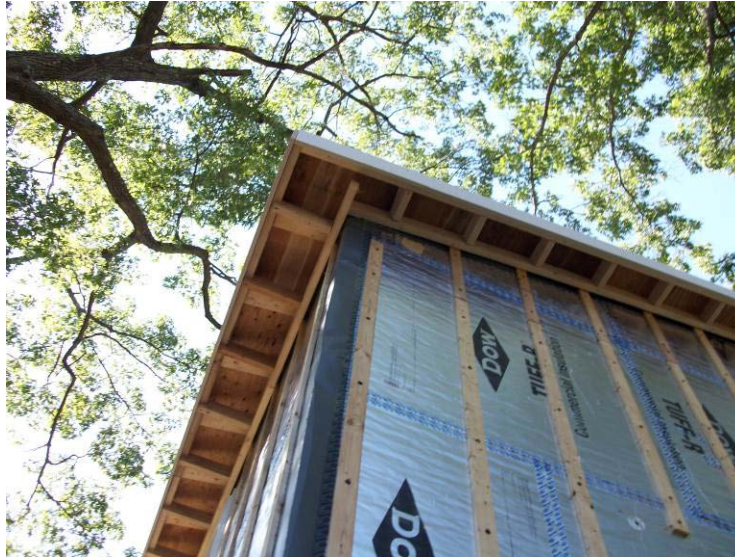
Figure 12. The Millbury Cape eave and rake overhang
