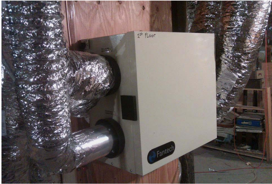
Figure 16. Somerville Triple Decker Fantech HRV. Photo used with permission from homeowner.
