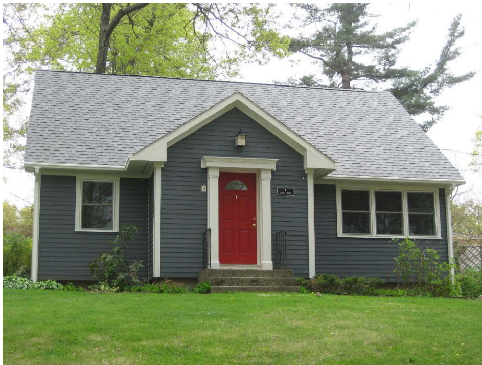
Figure 2. Post-retrofit Millbury Cape
