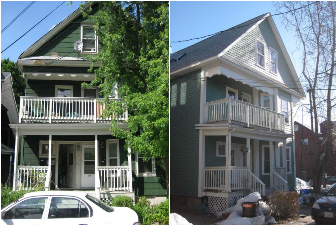
Figure 3. Pre- (left) and post- (right) retrofit Triple Decker located in Somerville, Massachusetts
