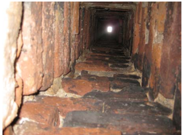
Figure 6: West chimney flue
