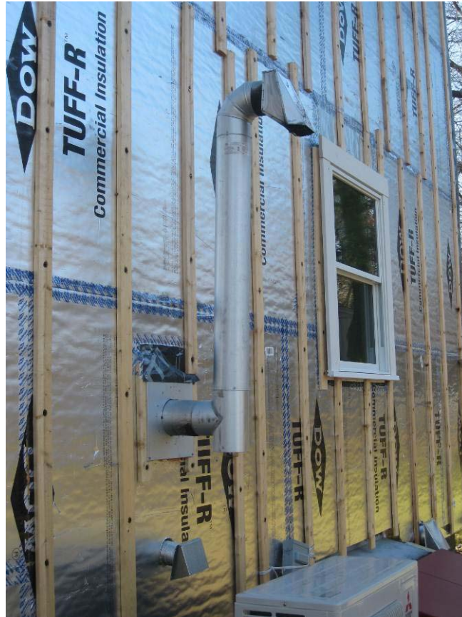
Figure 6. Insulating sheathing on the Millbury Cape
