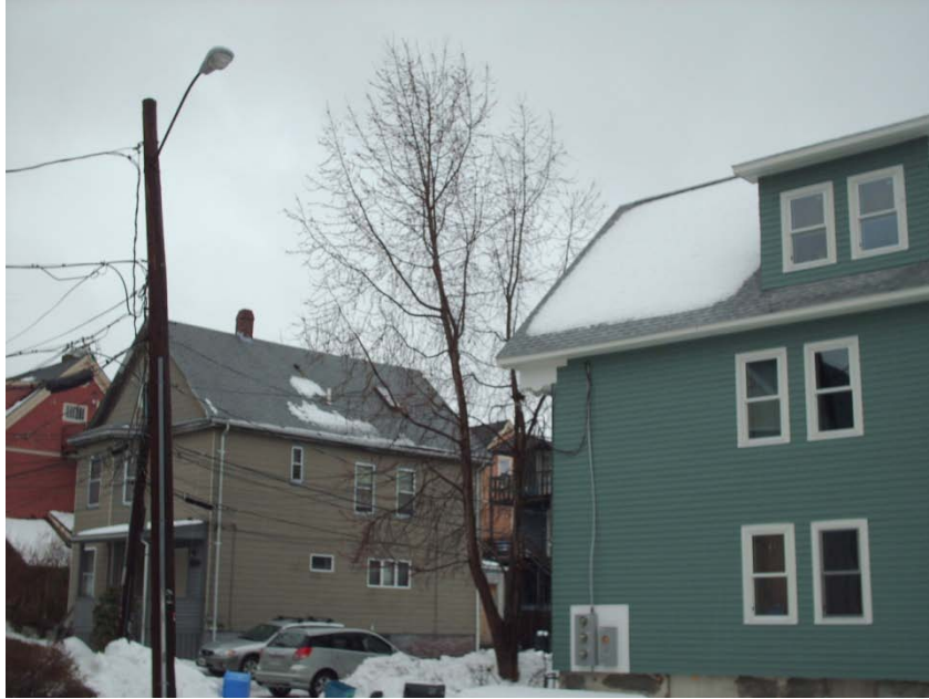
Figure 26. Post-retrofit Somerville Triple Decker, slow snow melting and no ice dams
