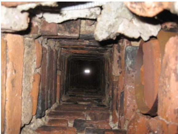
Figure 5: East chimney flue
