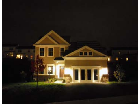
Figure 91. LED exterior lighting.
