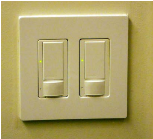
Figure 93. Manual on/automatic off control.
