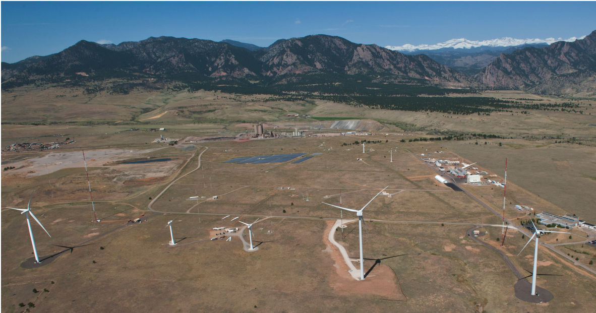
Figure 1. The view to the northwest across the NWTC in May 2011. Three utility-scale turbines are in the foreground of the picture to the left and right. The 38-m hub height Advanced Research Turbines are slightly set back. Photo by Dennis Schroeder, NREL/PIX 19018.
