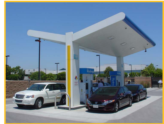
APC/Shell Pipeline station, Torrance, CA. Photo by Michael Penev, NREL
