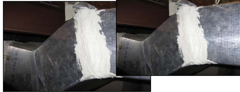
Figure 33. Sealing of duct shown in Figure 32 with mastic and fiberglass mesh.
