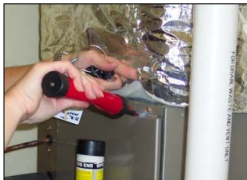
Figure 23. Using smoke to visually identify leaks at an air handler.
