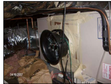
Figure 20. Airflow testing using a duct blower.
