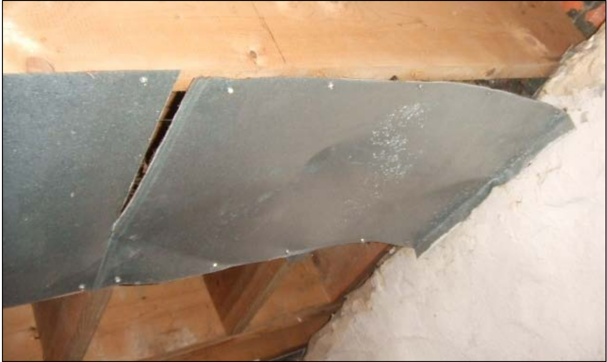
Figure 51. Floor joist bays used as panned returns.
