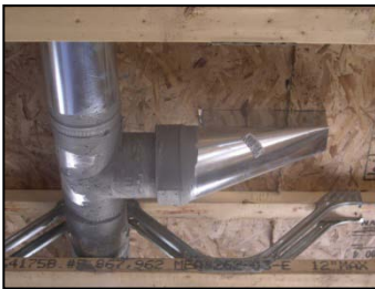
Figure 48. Sheet metal boot that has been sealed.
