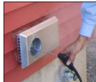
Figure 16. Testing CO levels at the exhaust flue of sealed combustion furnace.
