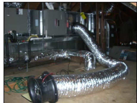
Figure 21. Duct leakage testing
