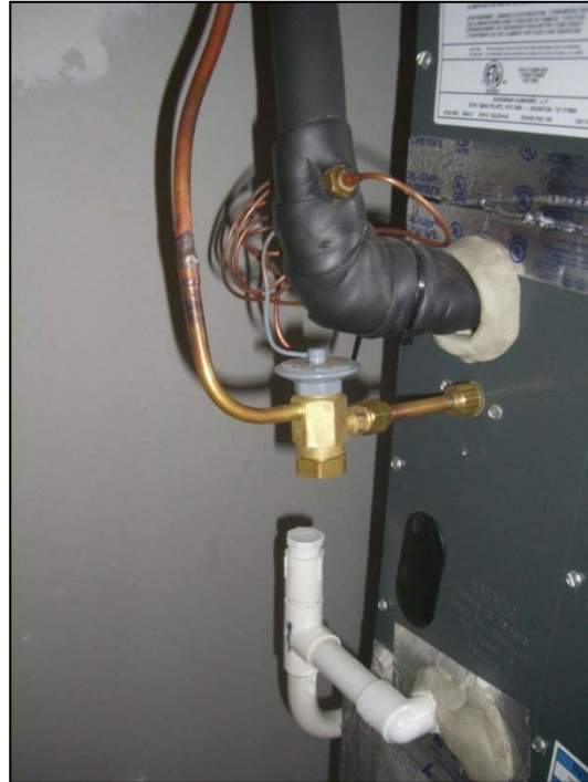
Figure 30. Plumber's putty installed around refrigerant piping to reduce air handler leakage.
