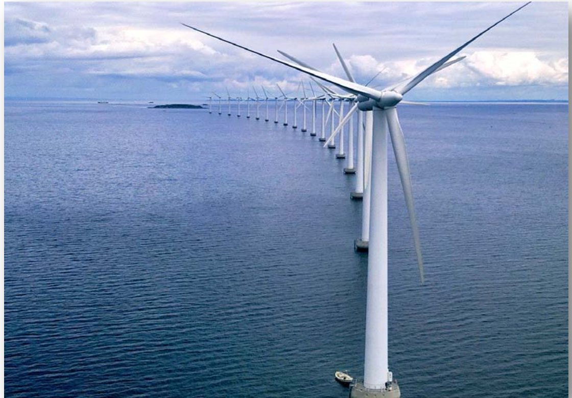
Photo from HC Sorensen, Middelgrunden Wind Turbine Cooperative, NREL/PIX 17855
