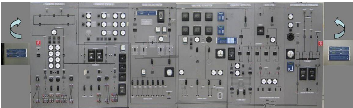
Figure D7.1 Photograph of Laboratory Simulator with new SEL Equipment Installed.
