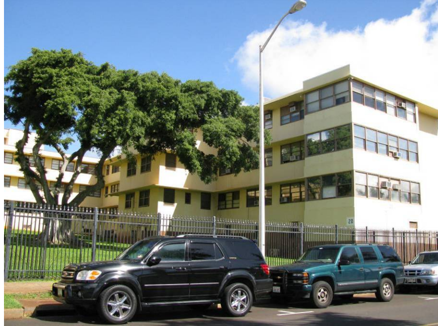
Figure D 12. Building 2D South Wall
