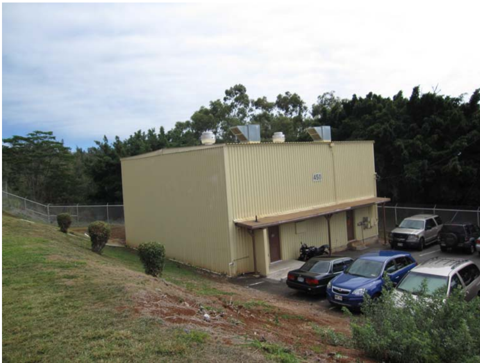
Figure D 44. Building 450
