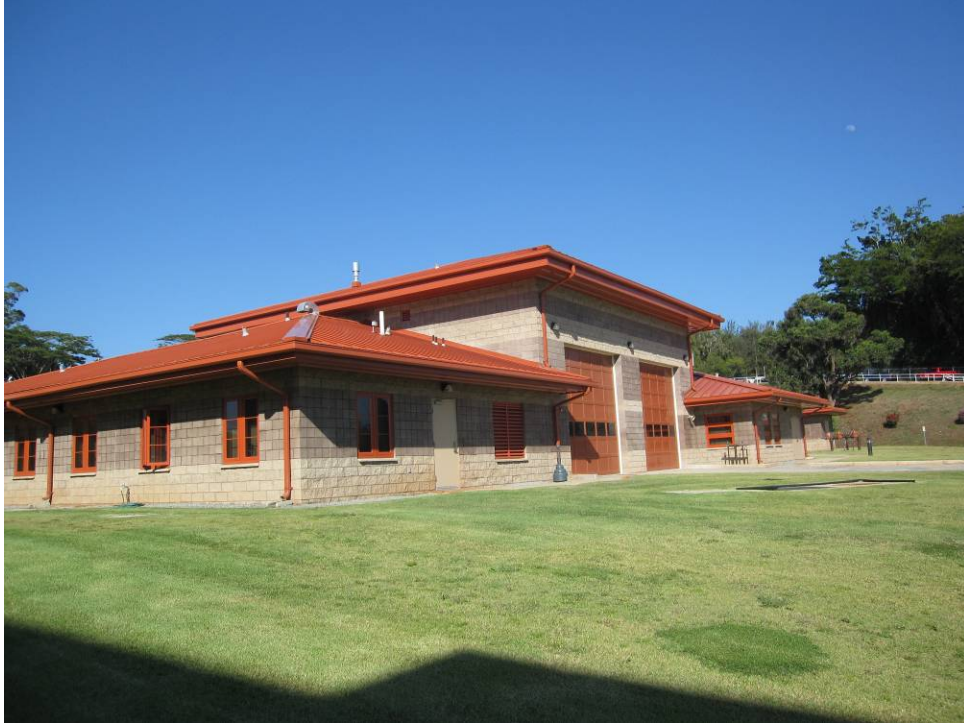
Figure D 42. Building 612
