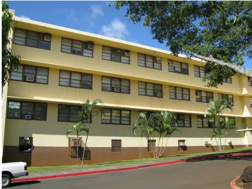
Figure D 11. Building 2D North Wall
