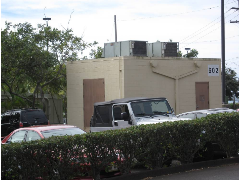
Figure D 36. Building 602
