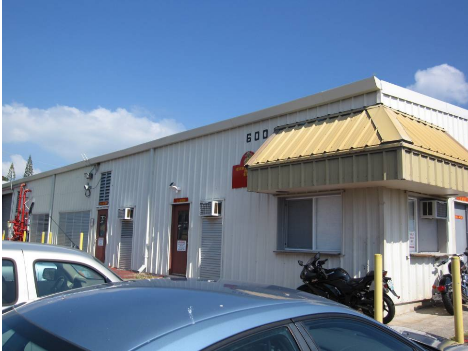
Figure D 34. Building 600
