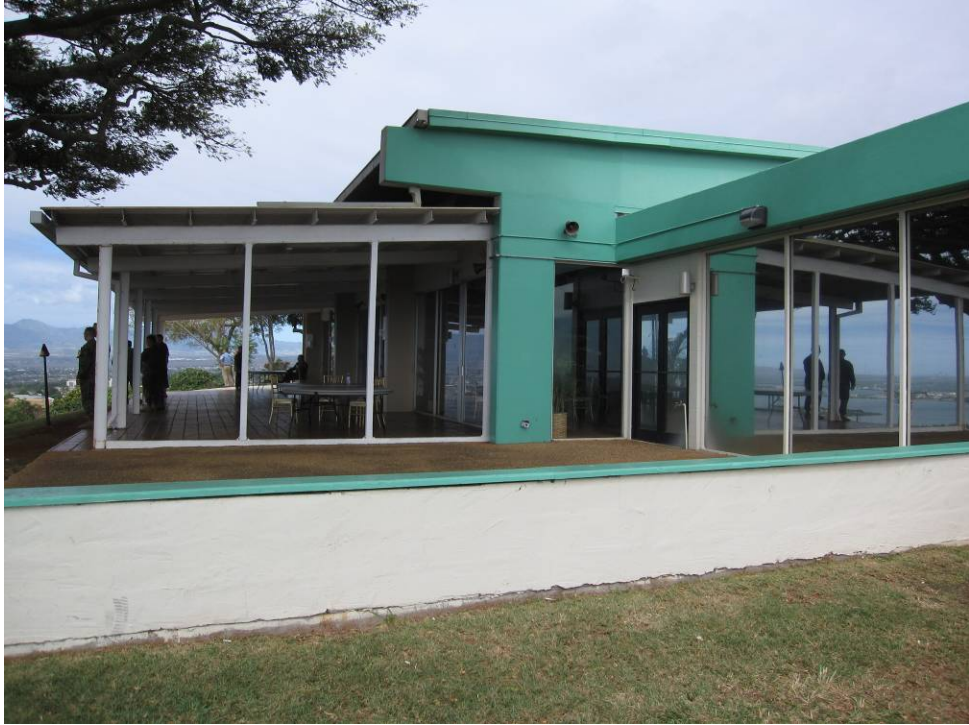
Figure D 40. Building 500, Rear View
