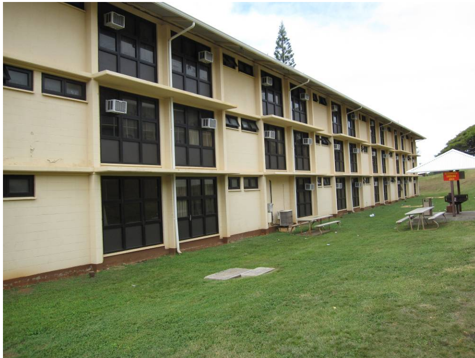
Figure D 33. Rear of Barracks 402
