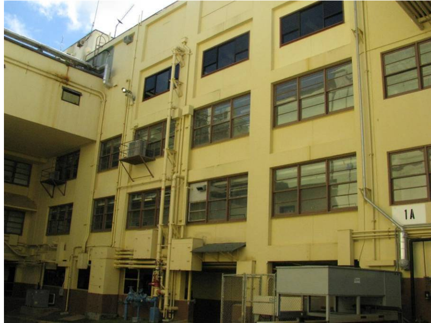
Figure D 6. Building 1A North Wall with Hallways Along Exterior Wall.
