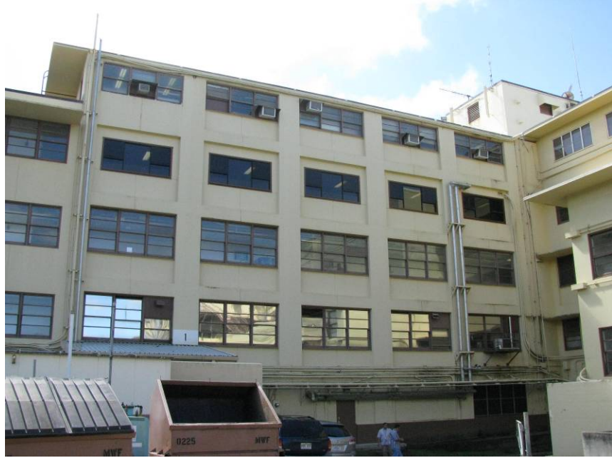
Figure D 3. Building 1 Rear View
