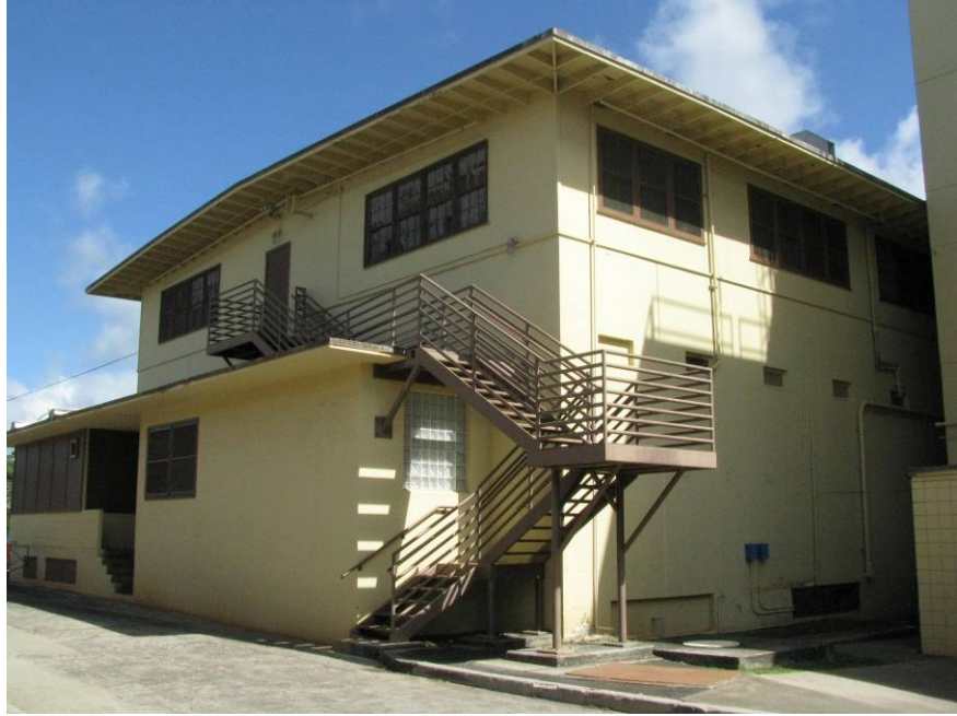
Figure D 21. Building 4 Rear View
