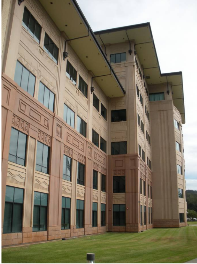
Figure D 30. Rear side of Building 700
