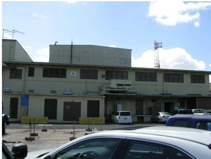
Figure D 20. Building 4
