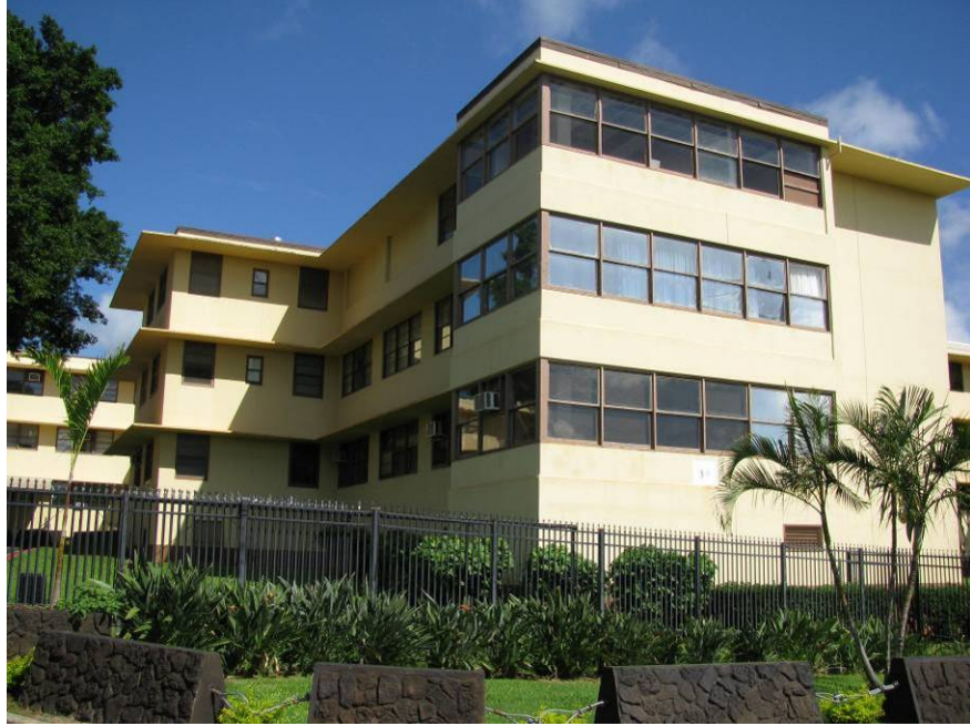
Figure D 15. Building 3A East Wall.
