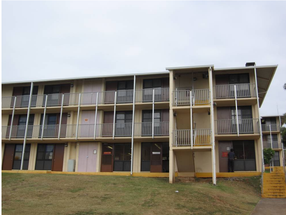
Figure D 32. Front of Barracks 402
