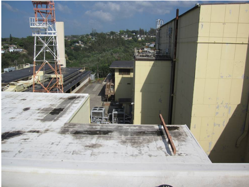
Figure D 25. Building 80 (right side) and Building 5 (left side)
