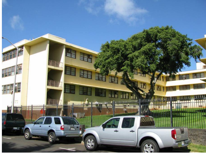
Figure D 9. Building 2C North Wall
