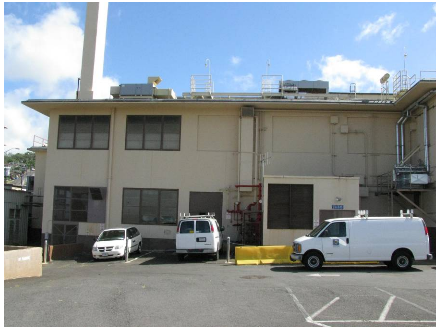
Figure D 23. Building 5 Exterior View
