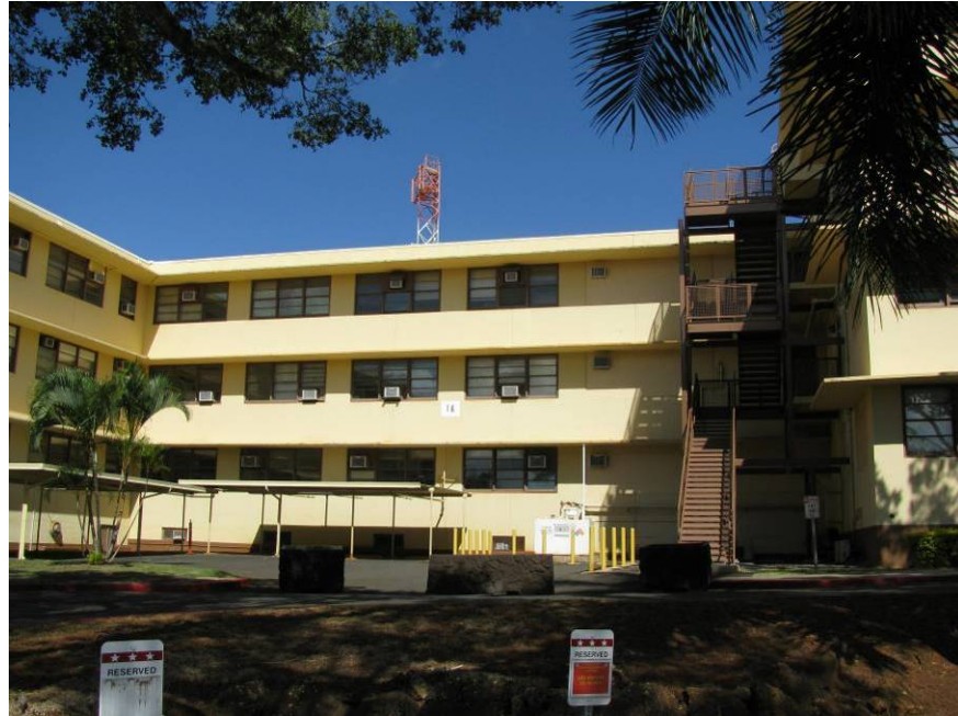
Figure D 5. Building 1A South Wall Showing Office Suites with Window Units
