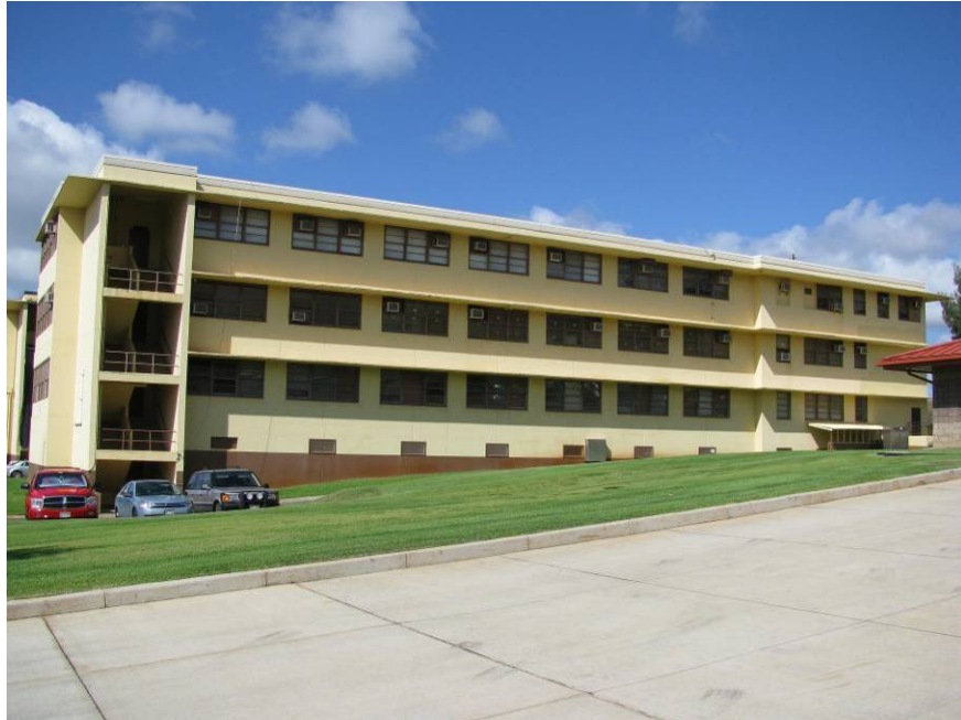
Figure D 17. Building 3B North Side
