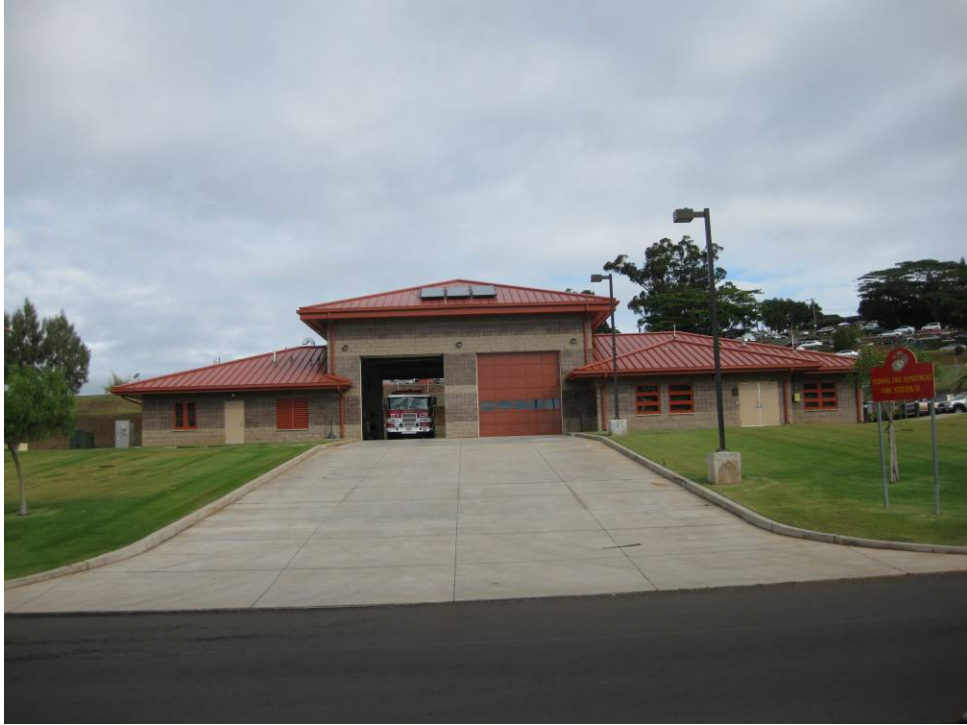
Figure D 43. Building 612 with Solar Hot Water System on Roof.
