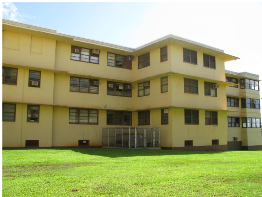
Figure D 18. Building 3B South Wall
