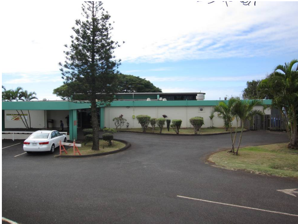
Figure D 39. Building 500, Front View
