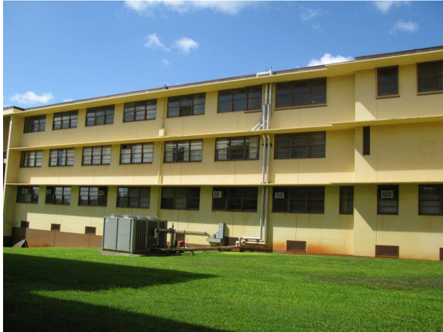
Figure D 14. Building 3A North Wall.
