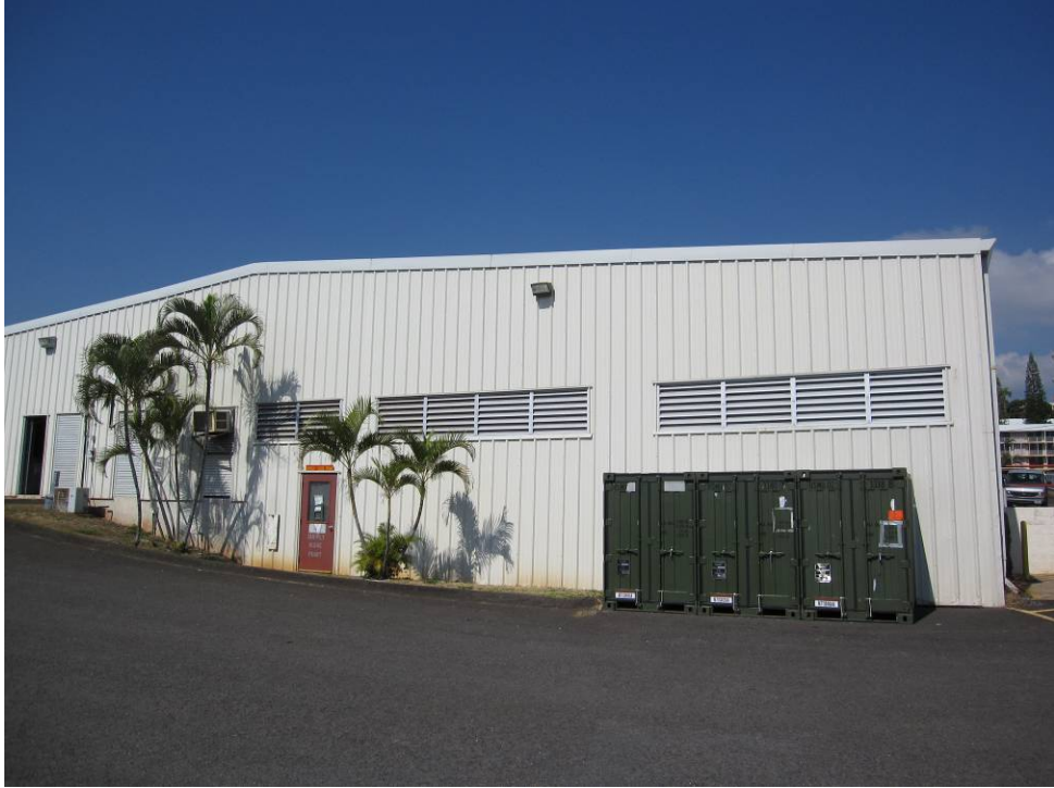
Figure D 35. Building 600 End View
