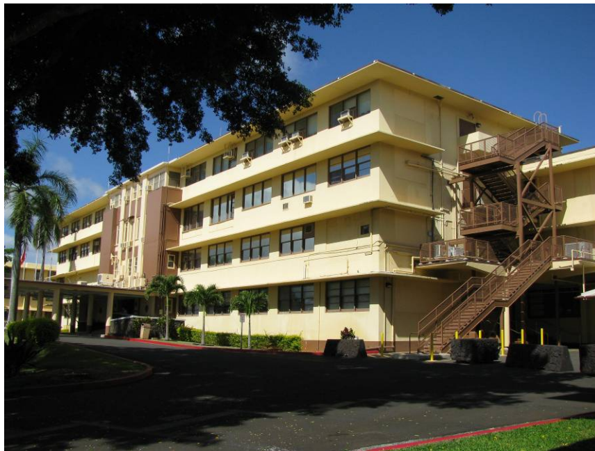
Figure D 2. Building 1 Front Side Main Entrance
