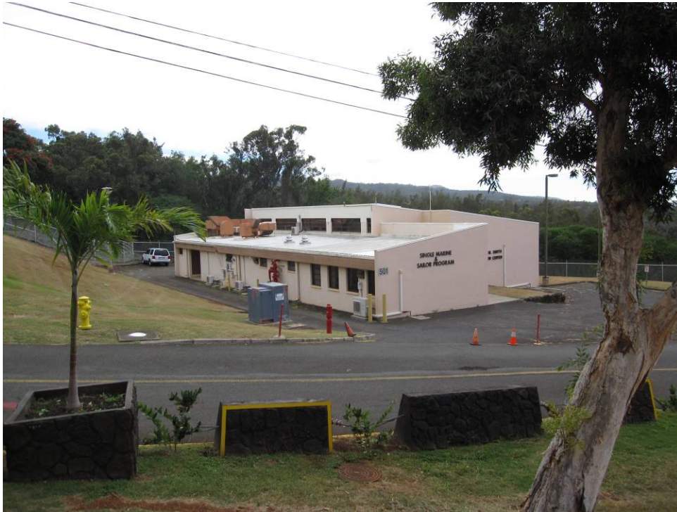
Figure D 41. Building 501.
