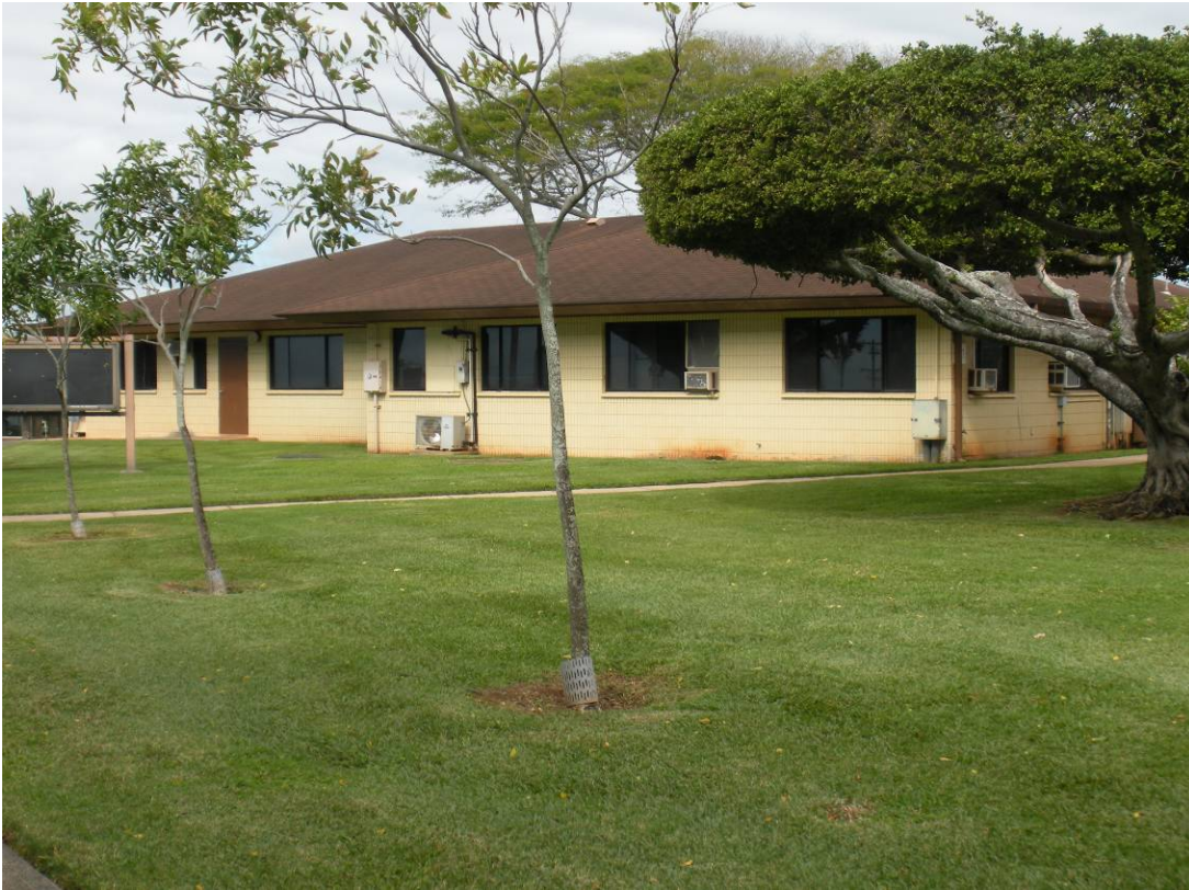
Figure D 38. Building 601
