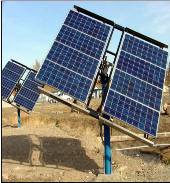
Figure E.1: Axis tracking PV array
