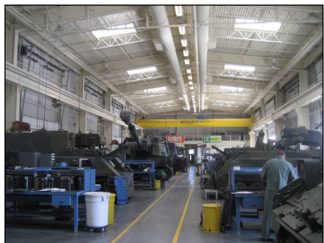
Figure E-5: Daylighting fixtures at the Yakima Training Center
