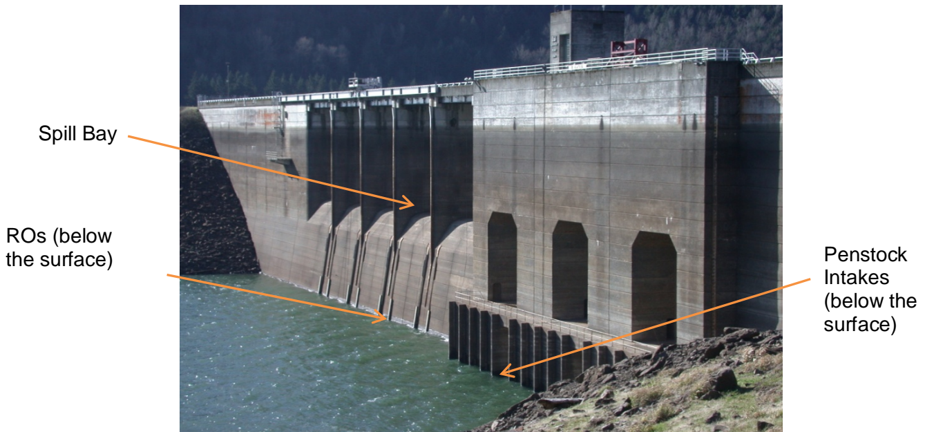
Figure 1.3. Upstream Face of LOP Showing Locations of the Penstocks, ROs, and Spill Bays
