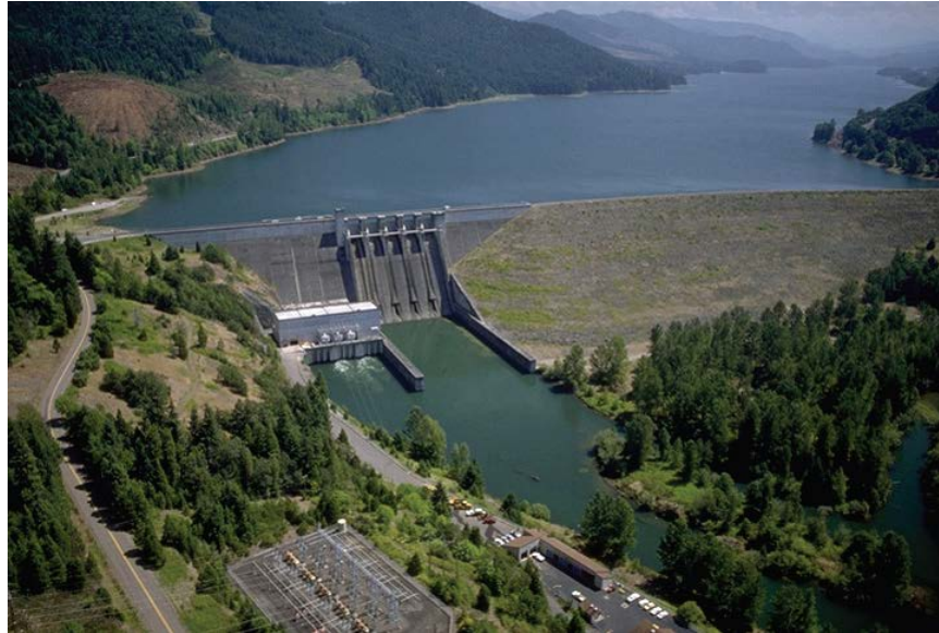
Figure 1.2. Aerial Photograph of Lookout Point Dam (courtesy of the USACE)
