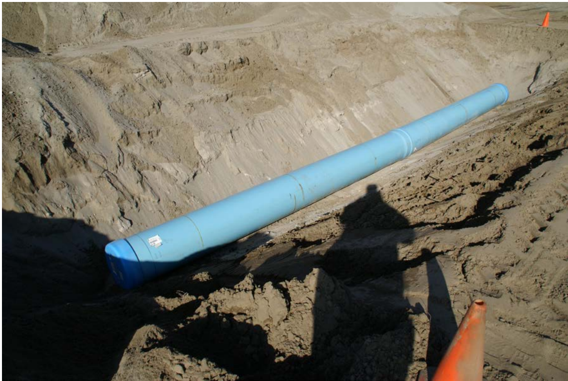
Figure 3.8. Empty 2-ft-Diameter × 40-ft PVC Pipe Buried 1.5 m with Ends Closed Off
