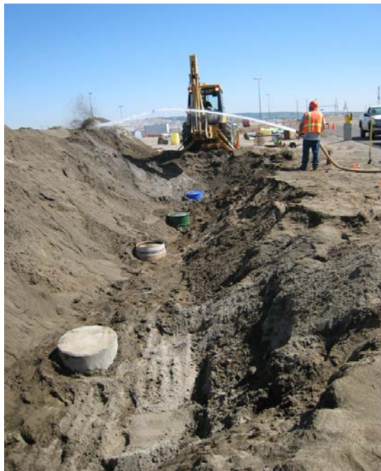
Figure 3.10. Four 55-Gallon Drums Buried Upright at Depth of 1.5 m (single depth)
