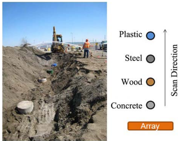
Figure 3.24. Scan Configuration for Targets #4–#7 Buried 55-Gallon Barrels
