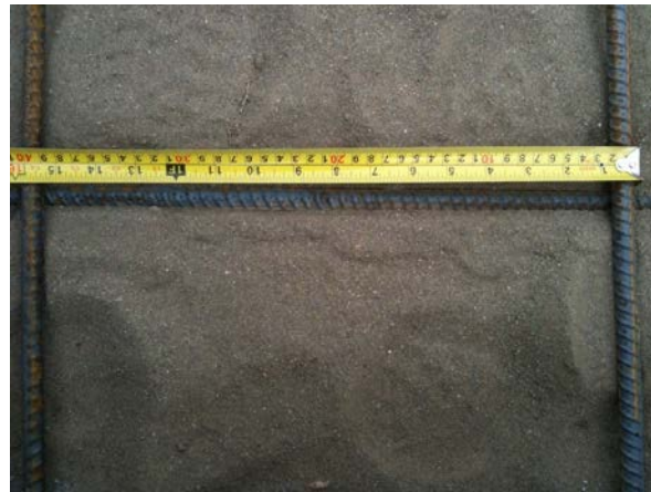
Figure 3.18. Photograph of 16-in. × 16-in. Grid Made of ½-in.-Diameter Rebar
