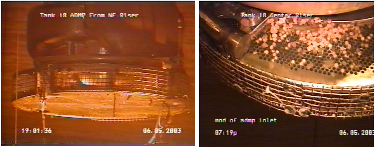
Figure 3-7. ADMP suction screen opening modification (post Tank 18-F installation).
