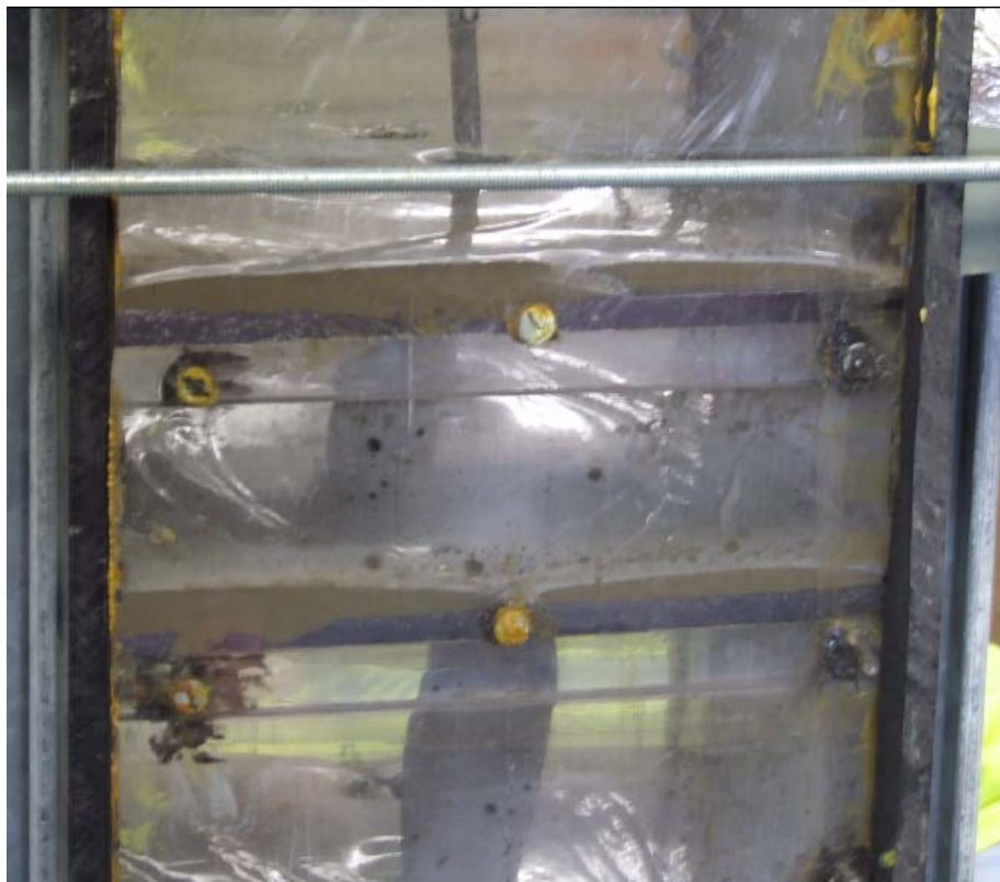
Figure 5-2. Tier 1A Test form being filled with Grout.
