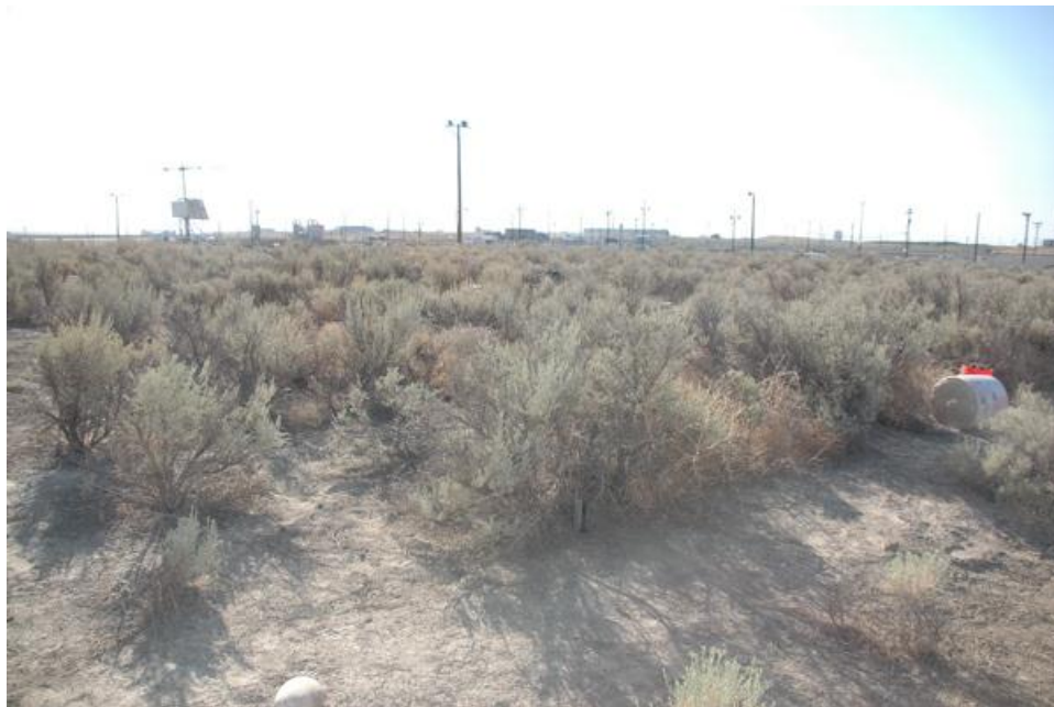
Figure 4.1. Prototype Hanford Barrier Cover Dominated by Artemisia tridentata in 2007, 15 Years After Establishment.
