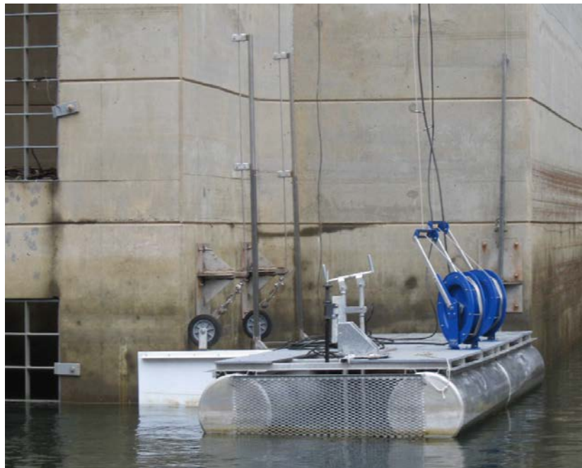
Figure 2.2. The Floating Platform (barge) Attached to the WTC Tower. The DIDSON and BlueView acoustic imaging cameras are 1.2 m below the water surface.
