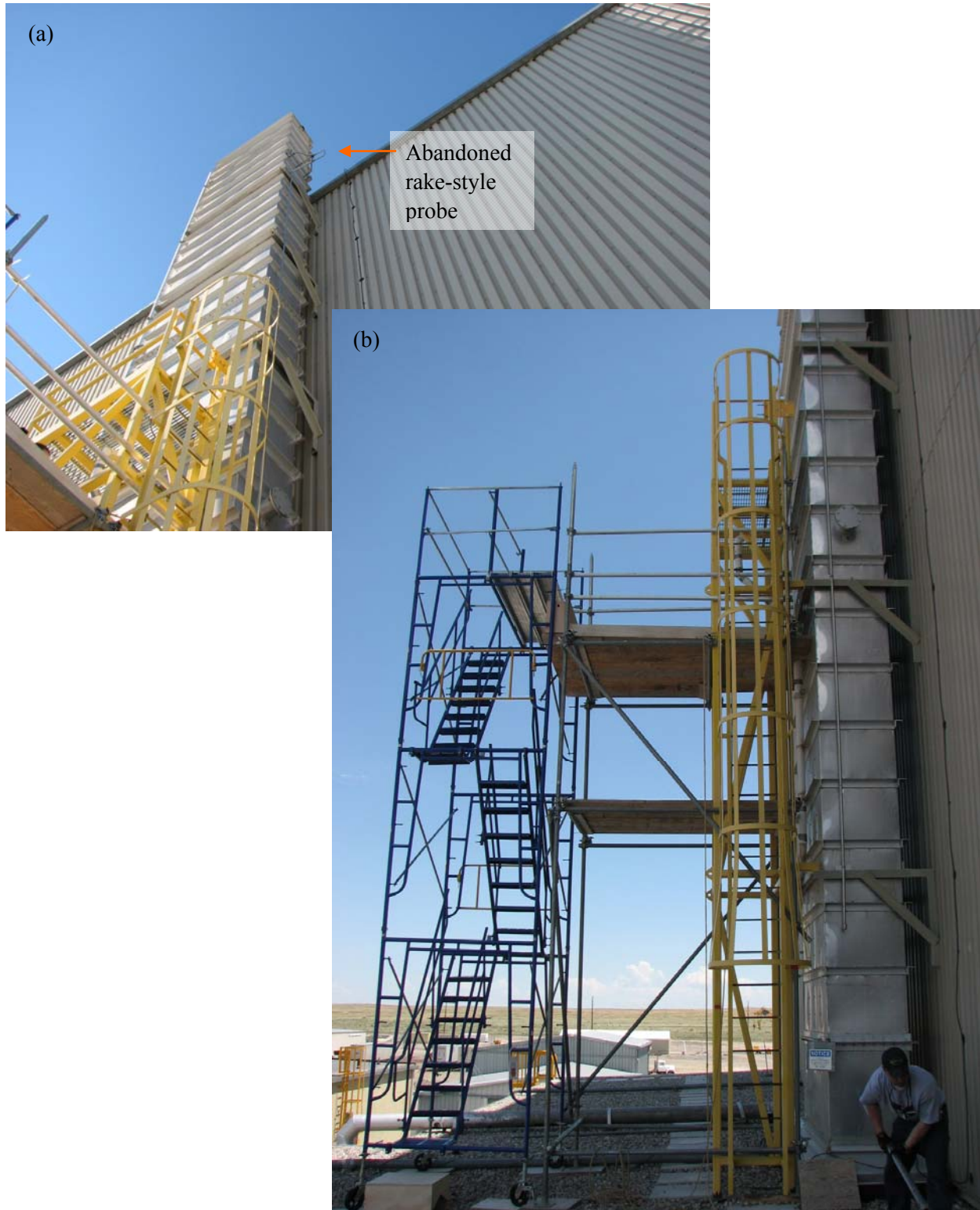
Figure 2.2. HFEF Building Exhaust Stack
