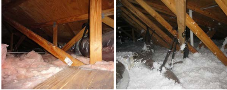
Figure K.9. Retrofit EH-03: Pre-Retrofit (left) and Post-Retrofit (right) Ceiling Insulation
