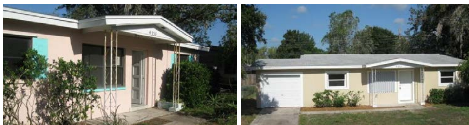
Figure K.17. EH-07 Pre-Retrofit (left) and Post-Retrofit (right)
