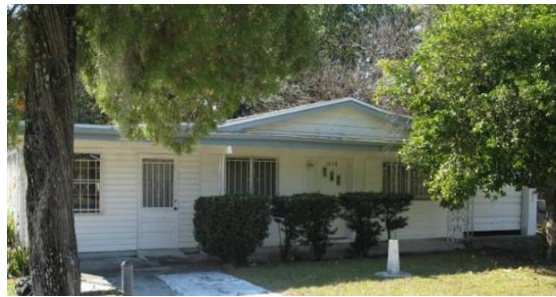
Figure K.1. EH-02 Pre-Retrofit (post-retrofit exterior unchanged)
