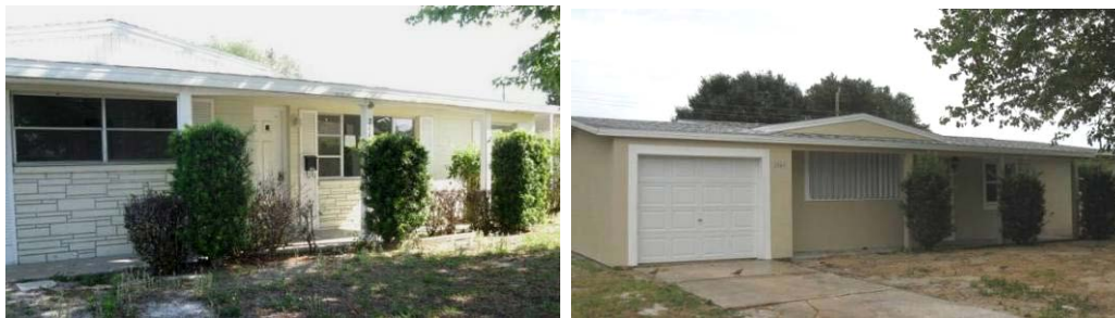
Figure K.14. EH-06 Pre-Retrofit (left) and Post-Retrofit (right)
