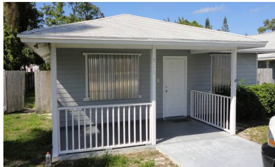
Figure K.5. EH-03 Pre-Retrofit with Hurricane Shutters in Place (exterior unchanged during retrofit)
