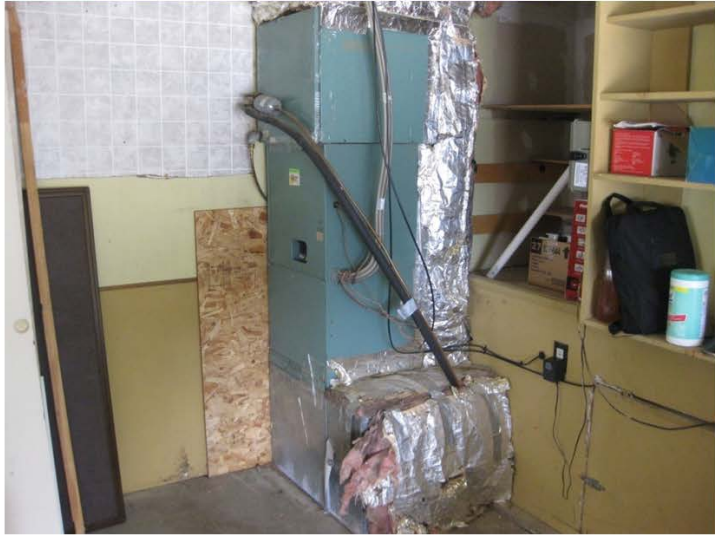
Above: air handler in the garage. Return air comes down a framed chase that is behind the air handler. The supply comes of the right of the air handler and enter the crawl space.
