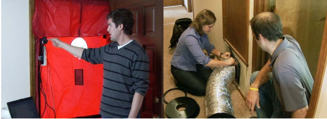
Figure 2.3. PNNL Research Staff Conducting a Blower Door Test (left) and Duct Blaster Test (right)
