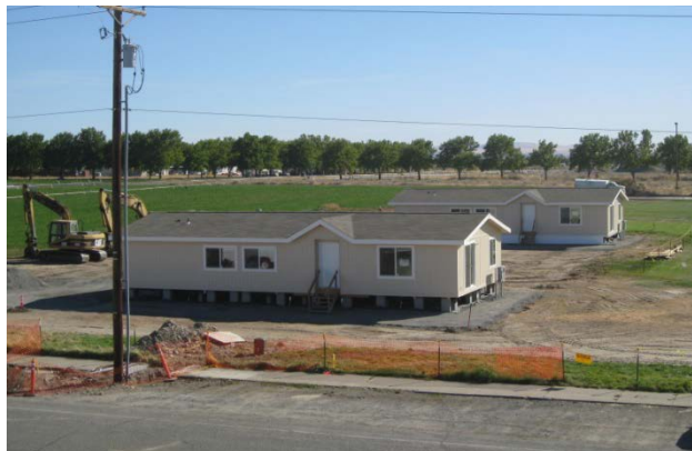
Figure 5.1. The Lab Homes During Setup in Late September 2011. The home in the foreground is the experimental home and the other is the baseline home.
