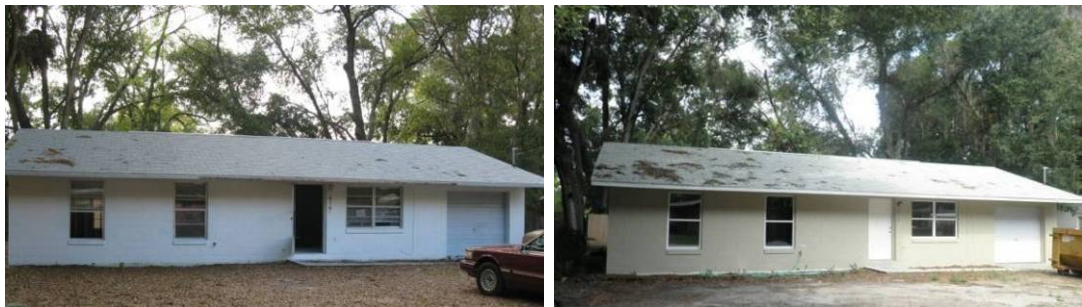
Figure K.10. EH-4 Pre-Retrofit (left) and Post-Retrofit (right)
