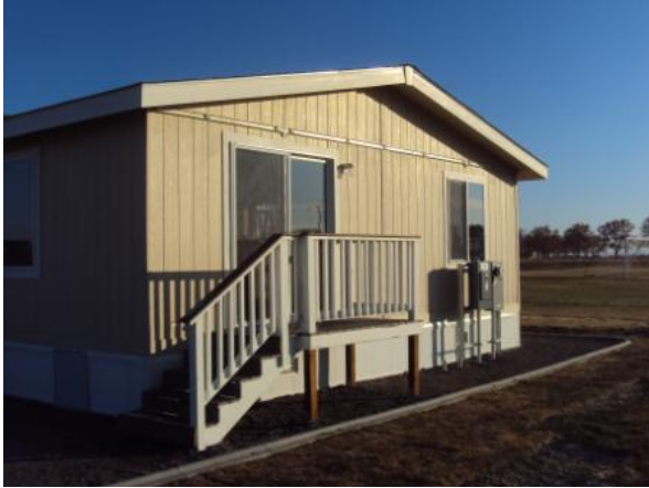
Figure 5.5. West End of Baseline Home. Note conduit tray (above slider and window) to hold exterior thermocouple wiring.
