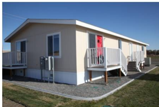
Figure 5.2. The Experimental Home in November 2011 Undergoing a Blower Door Test
